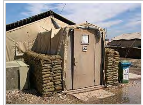
U.S. Army tent with constructed wooden entrance, air conditioner, and sandbags for protection. Victory Base, Baghdad, Iraq (April 2004).
