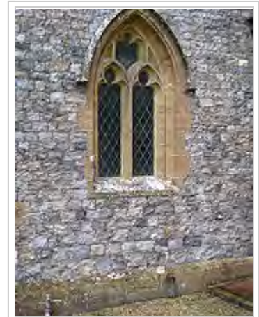
A flint church - the Parish Church of Saint Thomas, in Cricket Saint Thomas, Somerset, England. The height of the very neatly knapped flints varies between 3 and 5 inches (7.6 and 12.7 cm).
