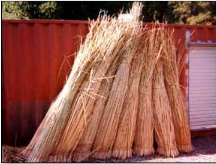
Eight 8-foot tule mats ready to be tied onto the house frame.
