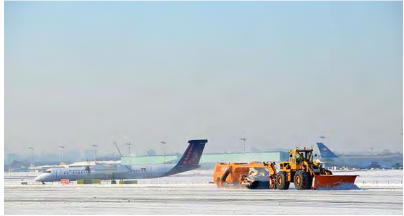
Airport snow-clearing operations include plowing and brushing.
