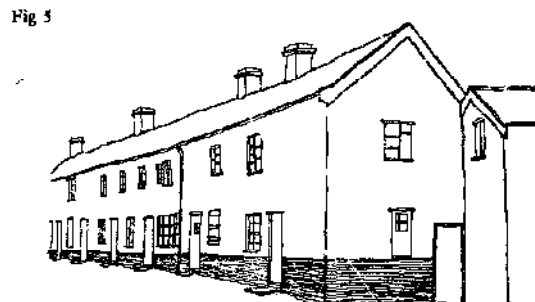
Fig 5 A row of clay lump cottages in Norfolk with a flint base and tiled roof.
