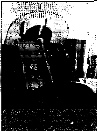
Fig 8. 'Solar kitchen, designed by J. Swet for Community Technology, Inc., Washington, D.C., developed to show that high temperature heat from the sun can be used indoors even when the sun is not shining. 'The glass-enclosed pipe is heated by solar radiation concentrated onto it by the trough-shaped reflector. An insulated extension (hidden by the enclosure far end) delivers the heat to the hotplate (partially hidden) on which the coffee pot and an as yet unbuilt thermal storage mass sit. The collector tracks the sun automatically. Larger versions could be developed for community-scale food processing or local light industries.' (From Hess).
