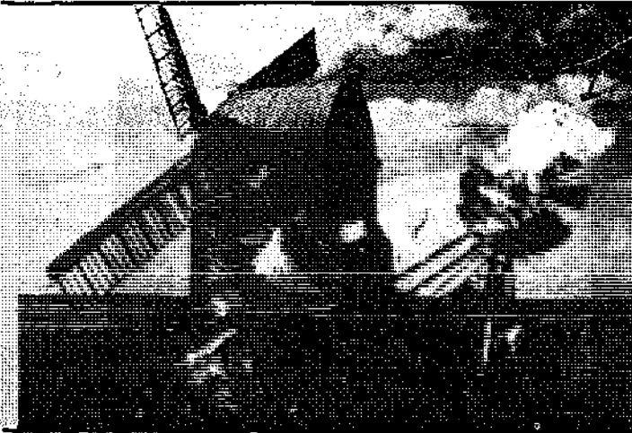
Fig 13. Traditional Windmills. (Upper left) Great Chishill post-mill, Cambridgeshire, oriented by a fantail. (Lower left) Chesterton tower-mill 19th century photograph of a unique structure, possibly designed by Inigo Jones: oriented by a winch inside the cap. (Below) Dutch 'Waterwipmolen': a drainage post-mill oriented by a capstan wheel. (Top right) 'Tjasker', smallest and simplest type of Dutch drainage mill lifting water by means of an Archimedian screw. (Lower right) A 'paltroek', a uniquely Dutch type, designed for sawing wood. The entire structure rotated on rollers on a brick base. (Far right) The most characteristic Dutch type, a thatched smock-mill oriented from the outside by a capstan wheel and spars attached to the cap.
