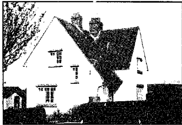
Chalk cement block house at Amesbury.
