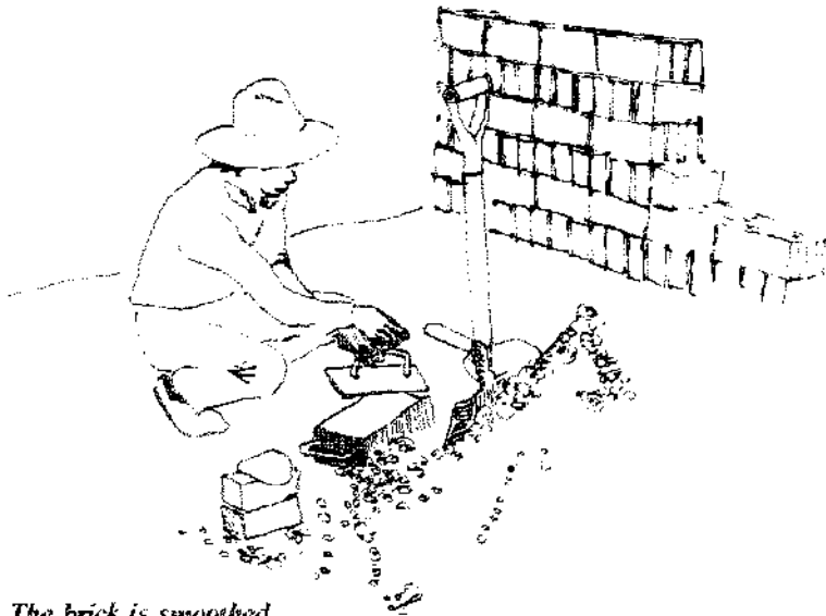
The brick is smoothed with a metal trowel.
