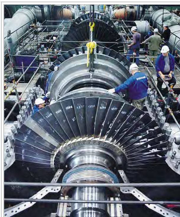
A steam turbine with the case opened. Most electricity is produced by thermal power stations with turbines like this one. Electricity consumption and living standards are highly correlated. [1] Electrification is believed to be the most important engineering achievement of the 20th century.
