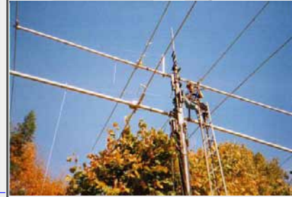
THE BIG TOWER NESTED ST 28 FT...MY SON MICHAEL WORKING FROM THE WORK TOWER, CHANGING ONE OF THE OMEGA MATCHES
