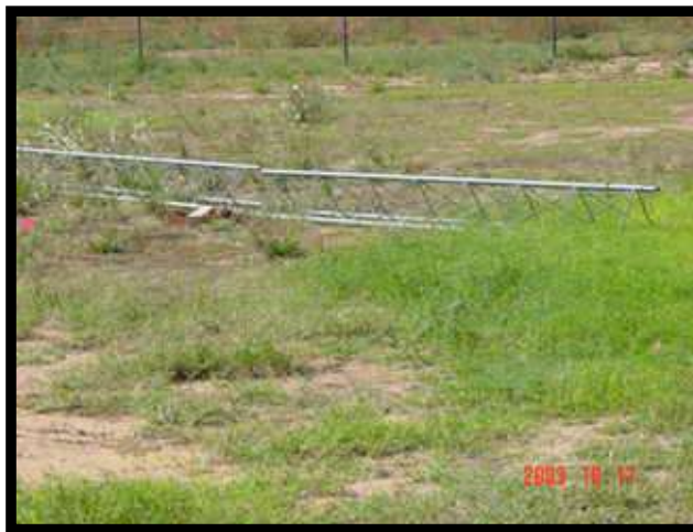
just south of the Crank up tower (see tower #1 page) Tower sections moved to location.
