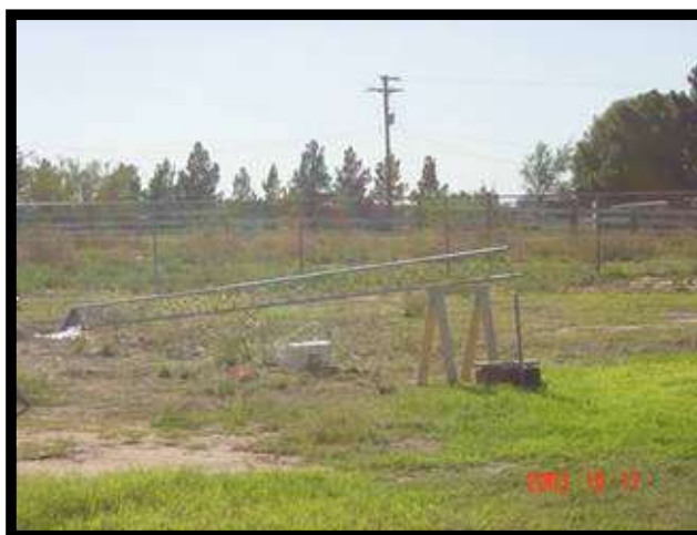
After getting ten feet up the section is laid over and another 20 feet added.
