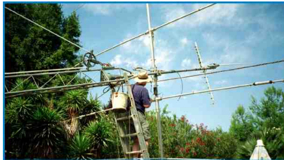
Art, K6XT does all the finishing touches to the assembly, here he is RTVing the Balun to weather proof it.
