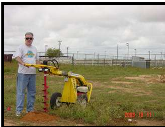
This is shot of project start.
