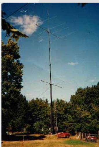
4X4 STACKS 30 FT BOOMS ON 2.5 TON FREESTANDING ROTATING TELESCOPING GK HB SKYNEEDLE
