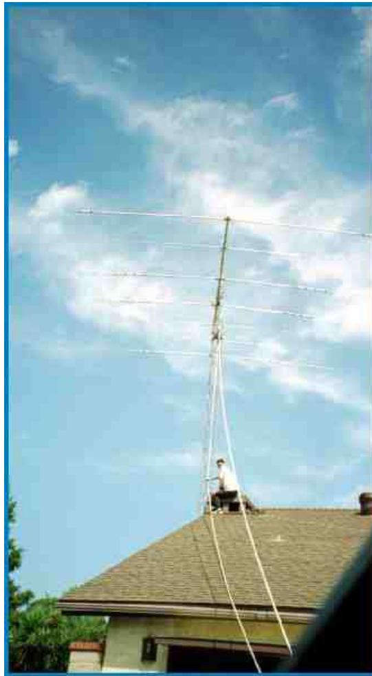
The Assembly is almost vertical now. Damon is getting ready to nest the tower into a roof eave bracket we made to hold it in place.
