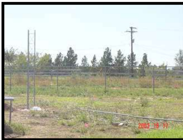
Hinged base. 1 st ten feet in place
