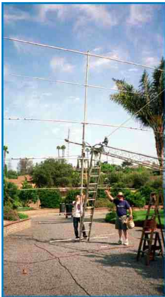
We used an extension ladder at the right height to support the tower and keep the antenna off the ground. The ladder is lashed to the tower and follows the tower as it is raised to this point.
