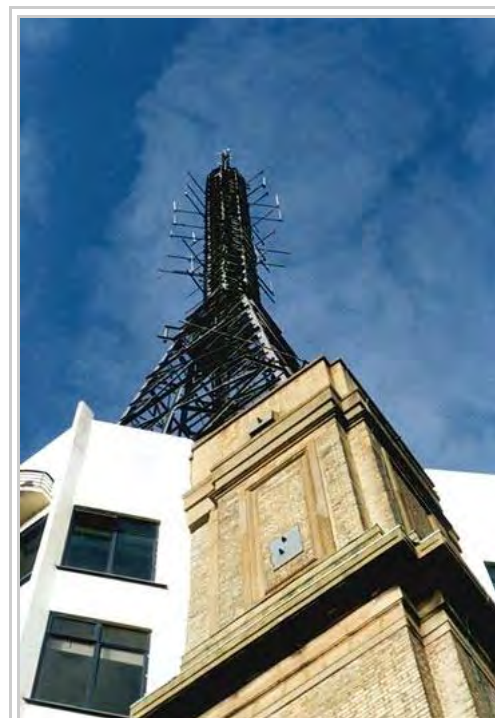
The Alexandra Palace, here: mast of the broadcasting station
