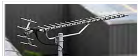
UHF television antenna on a residence. This type of antenna, called a Yagi-Uda antenna, is widely used at UHF frequencies.
