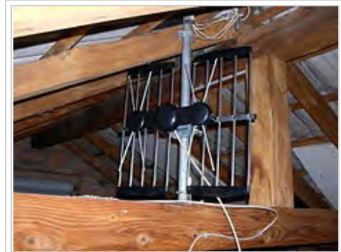
Another antenna type common at UHF; a reflective array TV antenna consisting of two high-bandwidth "bow tie" dipoles in front of a flat reflector screen.
