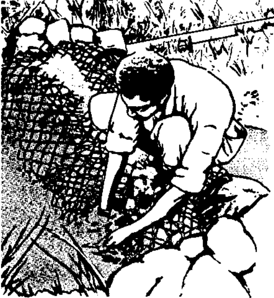
Building a gabion dam
