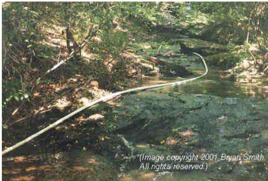
Figure 2. The 1-1/4 inch Schedule 40 PVC drive pipe supplying the ram pump. Note the curves in the pipe due to the geometry of the stream channel. The pump worked quite well despite the lack of straightness of the pipe.
