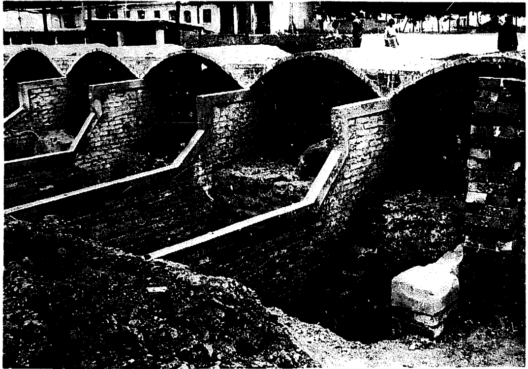
Fig. 2 Arch-shaped shelter for pigs with frontal pit. Ta Heh Production Brigade, Hebei Province.
