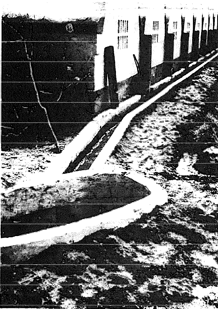
Fig. 32 Construction of a bio-gas plant, inlet on the right; outlet on the left in background. Cheng Hsiang Production Brigade, Jiangsu Province.
