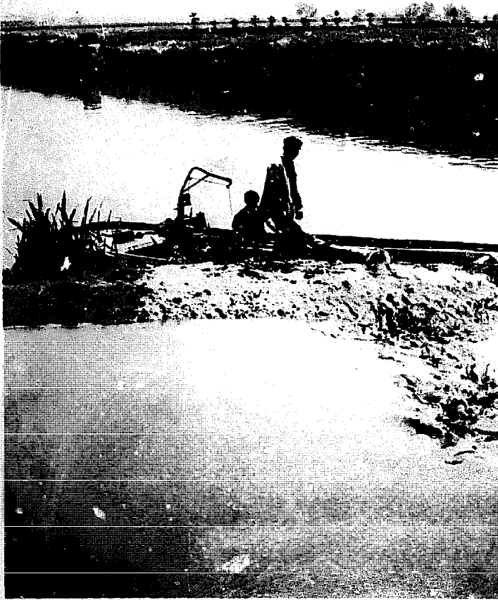
Fig. 6 Boat for sucking silt from the bottom of the canal. Foreground: Silt tank. Malu People's Commune, Shanghai
