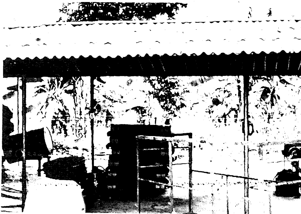
Fig. 12b Finished asphalted sheets in position.
