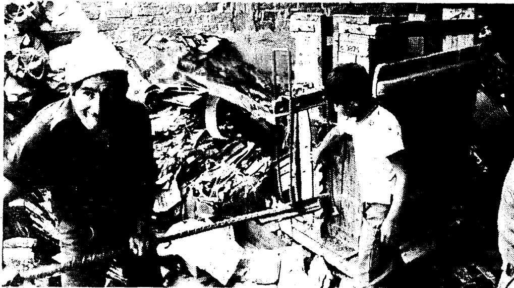
Fig. 6c The lever end is fitted under a low tooth and force applied. The hanger is slipped over the nearest tooth and the force is released. The operation is repeated at the other end, so that the hanger already in place can catch a lower tooth.
