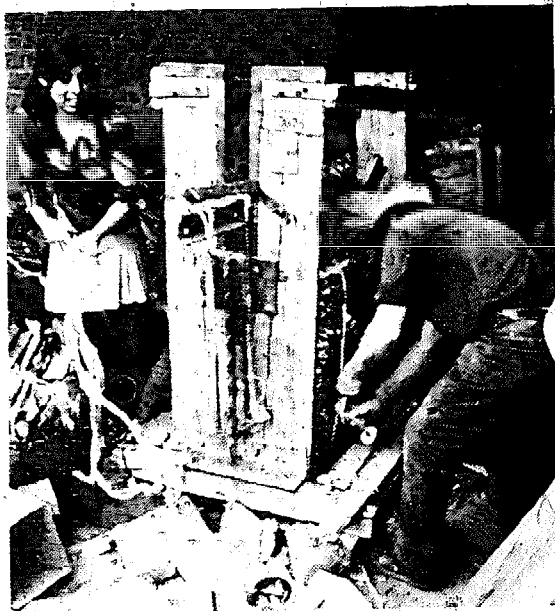
Fig. 6e Wires are inserted, using the long wiring needle, and twisted together.
