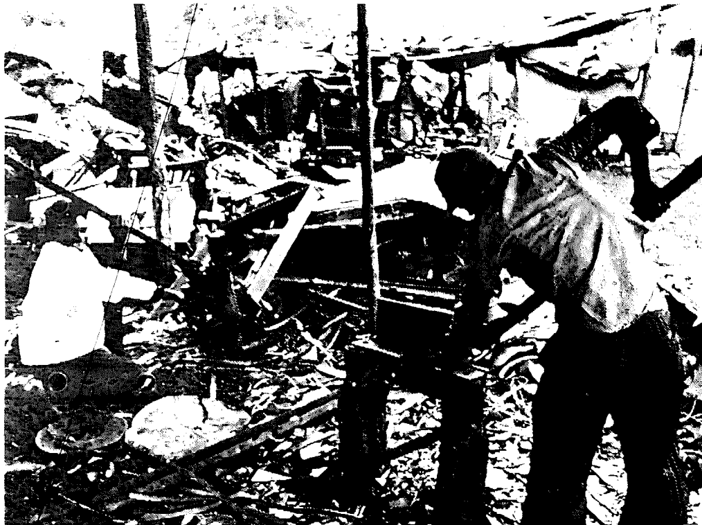
Fig. 20 Hand-made metal forming machines: this workshop included a shear, a punch, a bending machine and a machine for cropping reinforcing bars, all made with a hacksaw, hand drill, etc. Note how the machines have been mounted on wooden trunks, hammered into the ground in the absence of a concrete floor.
