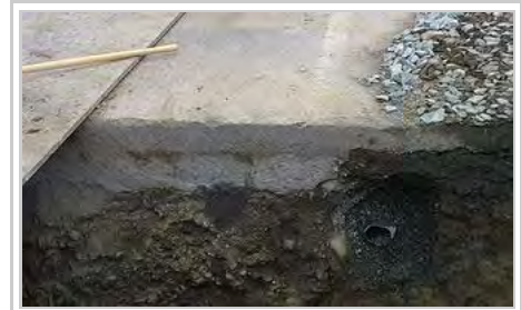
An example of composite pavement: hot-mix asphalt overlaid onto Portland cement concrete pavement
