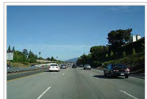
Concrete roadway in San Jose, California
