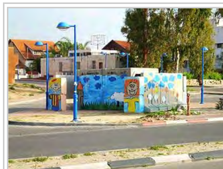
Entrance to a public bomb shelter in Sderot, Israel.
