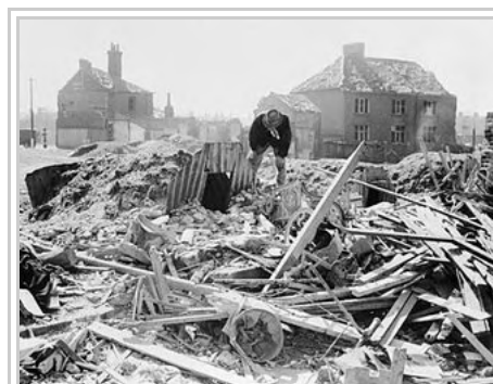
Two Anderson shelters standing intact amid a scene of debris in Norwich.
