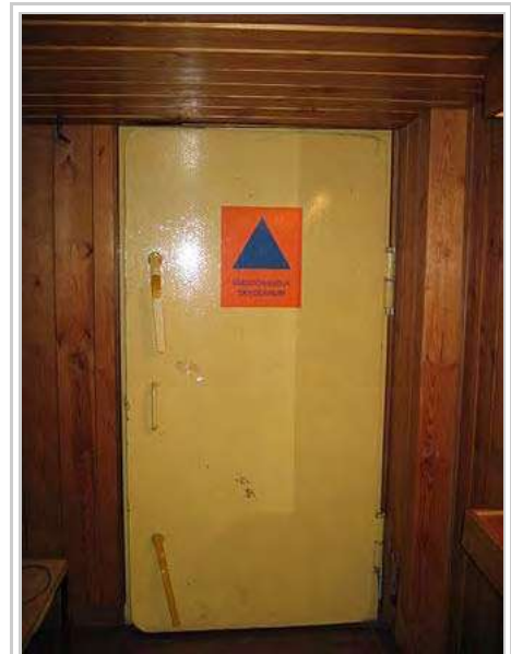
A normal Finnish S1-shelter steel door. S is short for suoja (protection, shelter).
