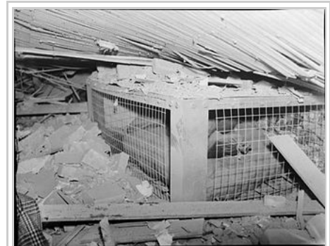
A Morrison shelter containing a dummy, after the house it was in had been destroyed as a test
