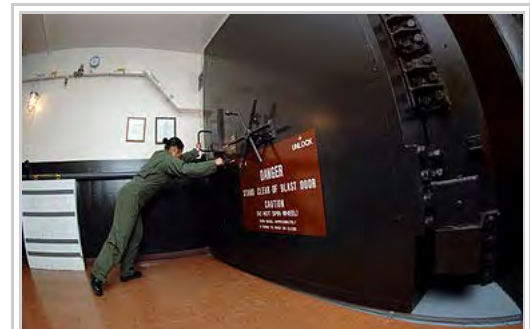
Blast doors in a missile control bunker at Minot Air Force Base, North Dakota.
