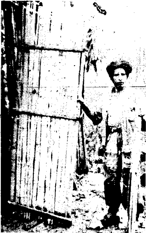
Figure 18.--A pioneer settler in eastern Peru has made his cabin door with material that came easily to hand--culms of a wild bamboo, Guadua sp.
