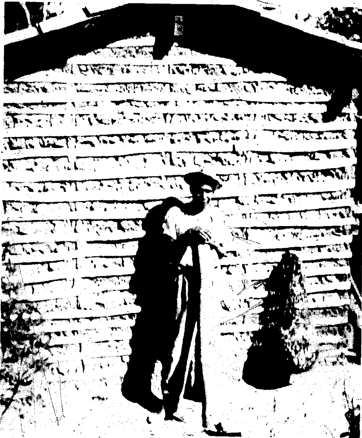
Figure 12.--Wide bamboo strips support and protect an adobe wall in El Salvador, forming a type of construction called bajareque in many Latin American countries. In El Salvador the common bamboo, Bambusa vulgaris , is available everywhere except in the driest areas, and its culms are standard material for many purposes.
