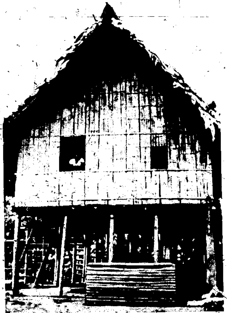
Figure 2.--From supporting posts to rafters and sheathing, this cottage in the Ecuadoran lowlands is made entirely of native bamboo, Guadua angustifolia . The posts may serve for five years; the siding may remain in serviceable condition for decades.
