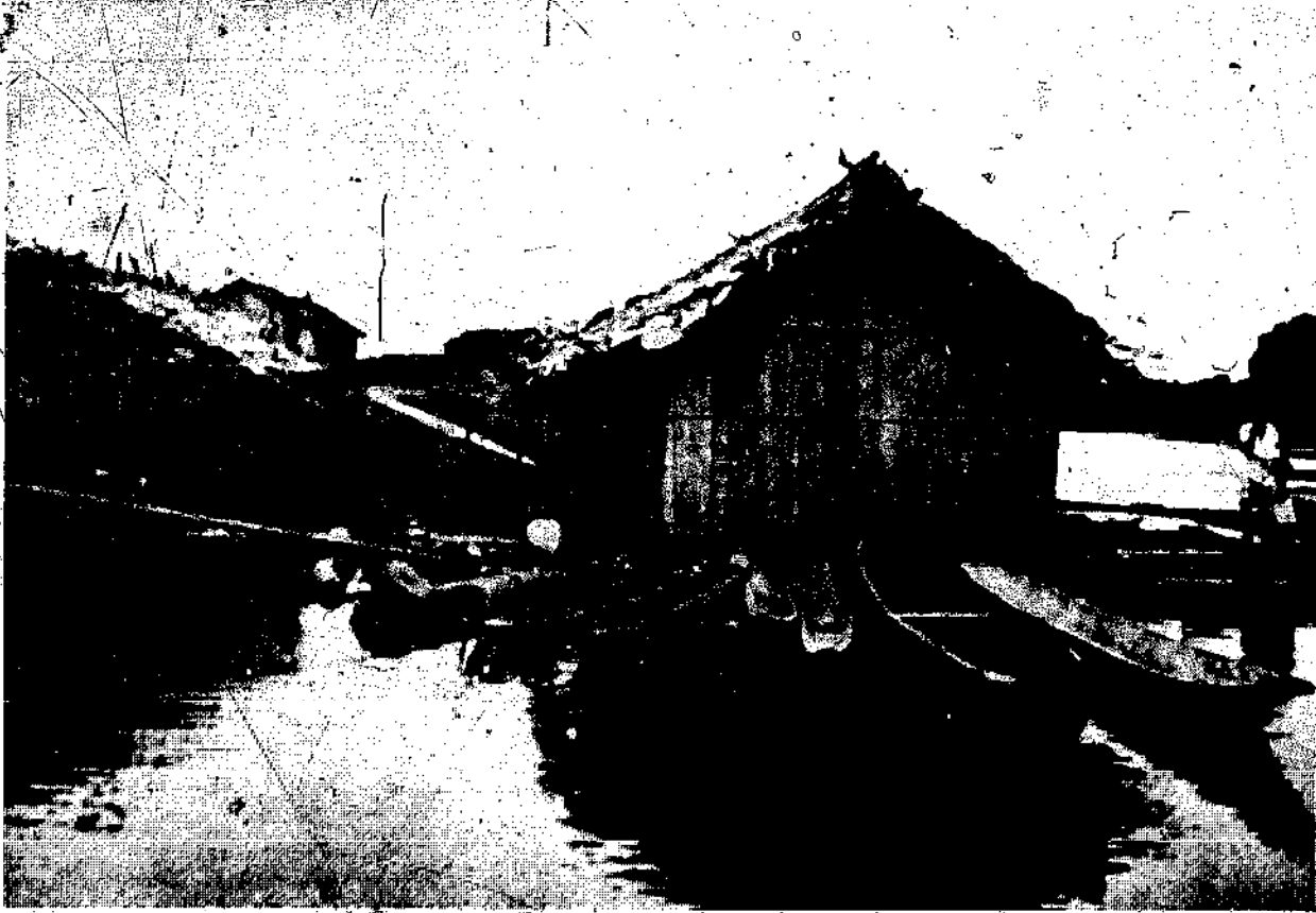
Figure 14.--Bamboo house, buoyed up by balsa logs, lies anchored in an Ecuadoran river. The walls are made of bamboo boards, and the leaf-thatched roof is held in place by bamboo riders resting across the comb..
