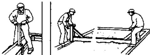
Figure 3.23 Manual compaction of foundation and floor slab.
