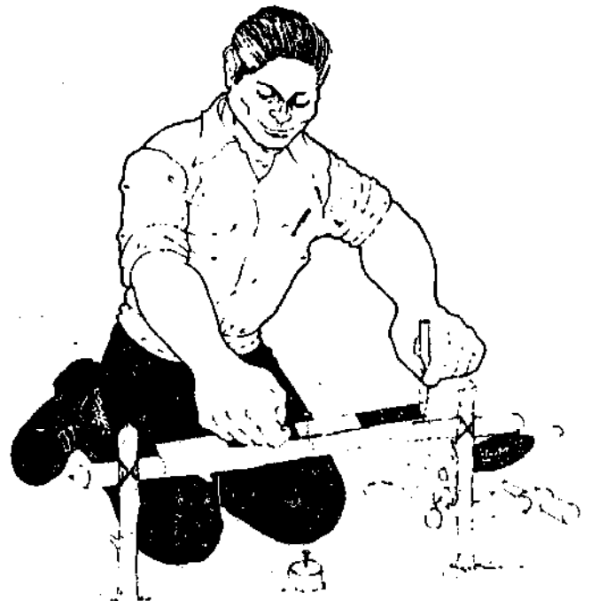
Using the nail as the center point, mark the width of the foundation on the batterboard.
