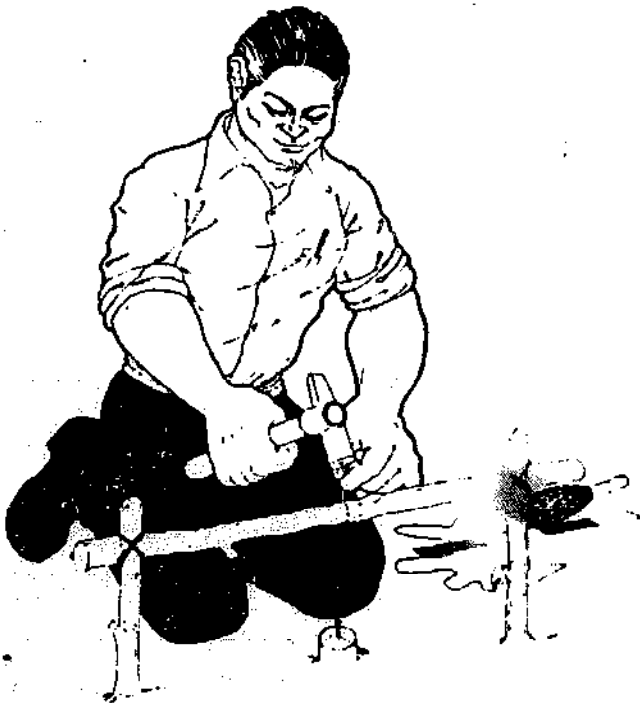
Put a nail in the batterboard at the mark.
