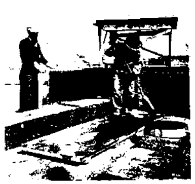
FORMS ARE DILED before use to permit removal as soon as ramming is complete. Concrete footing is scored to assure good water- and frost-proof bond with the wall.
