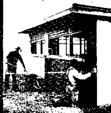
EXTERIOR SURFACING on Miller house consists of dagga-cement plaster brushed with water-proofing and finished with a cement base. No surface failures in this finishing to rest of new finish.
