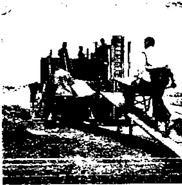
SOIL IS CARTED in wheelbarrows along ramps to point of ramming. This need for ramps and scaffolding sets practical limit of one story to use of rammed earth.
