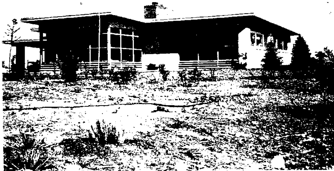
EXTERIOR SURFACING on Miller house consists of dagga-cement plaster brushed with water-proofing and finished with a cement base. No surface failures in this finishing to rest of new finish.
