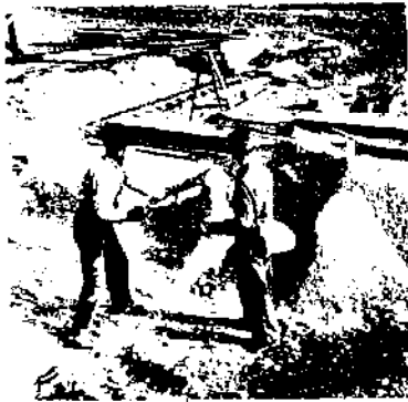
SOIL IS SIFTED through coarse mesh to remove stones and debris. Aggregates can range from fine sand up to large gravel but finer particles must predominate.
