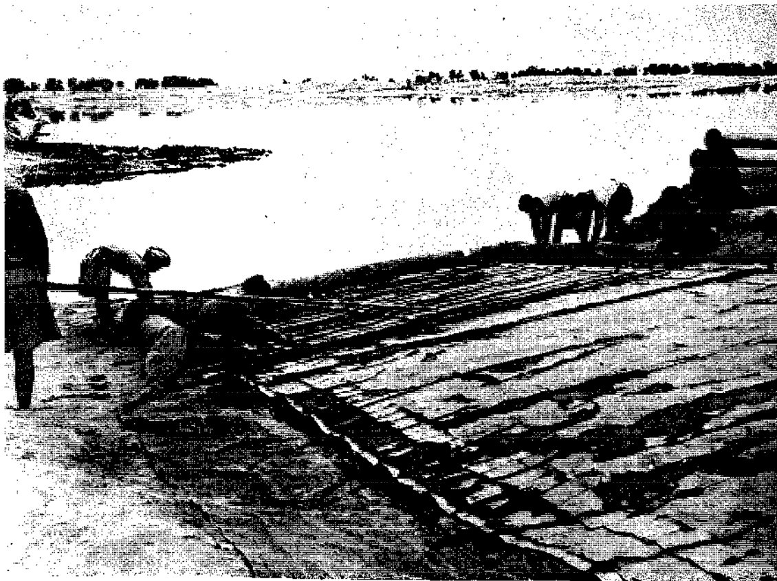
Photo 1. Bamboo inserted into the matbridge.
