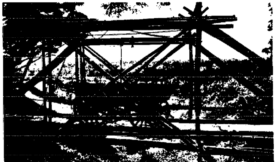
The Bridge under a 3,500-pound Load
