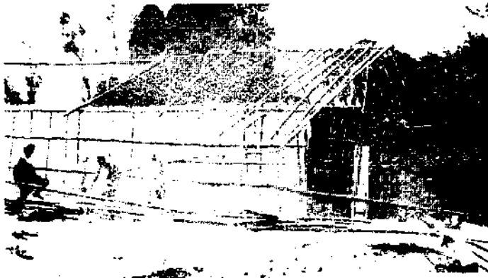
5. Placing bamboo poles to form the roof frame.
