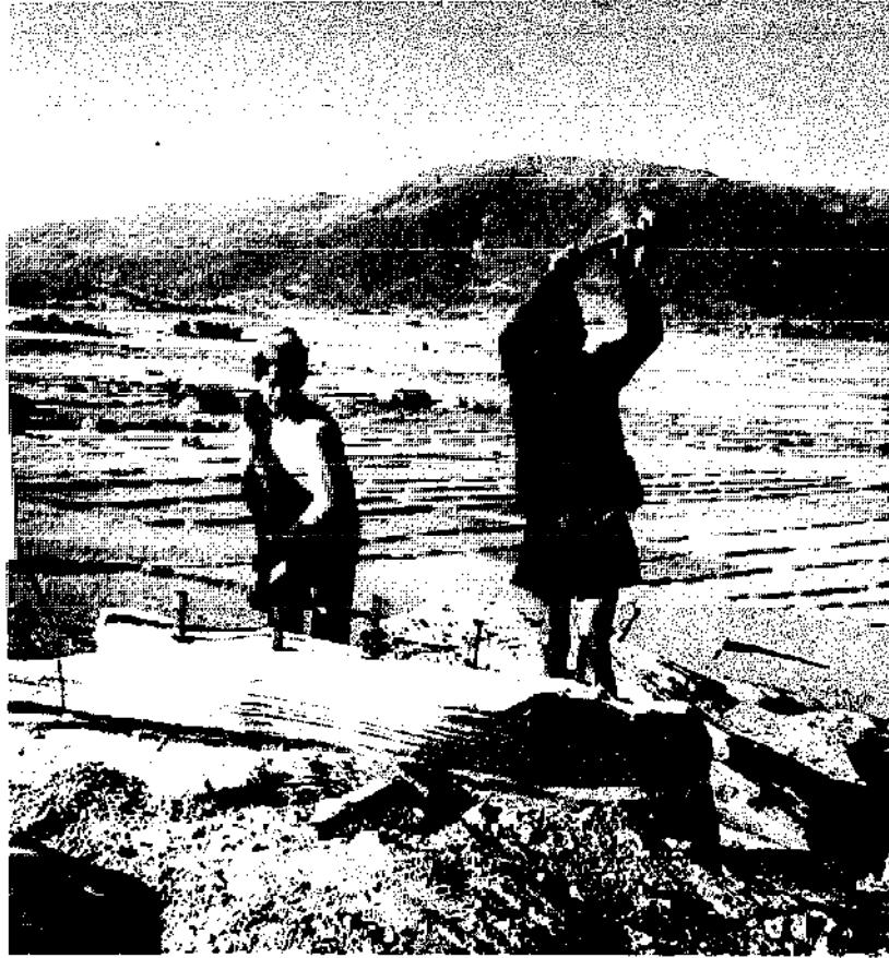
Above: Wedges are inserted into sandstone then split with sledge-hammers in Nepal. Below: Splitting sandstone, first with a hammer and chisel (left) then with a sledge-hammer peen.
