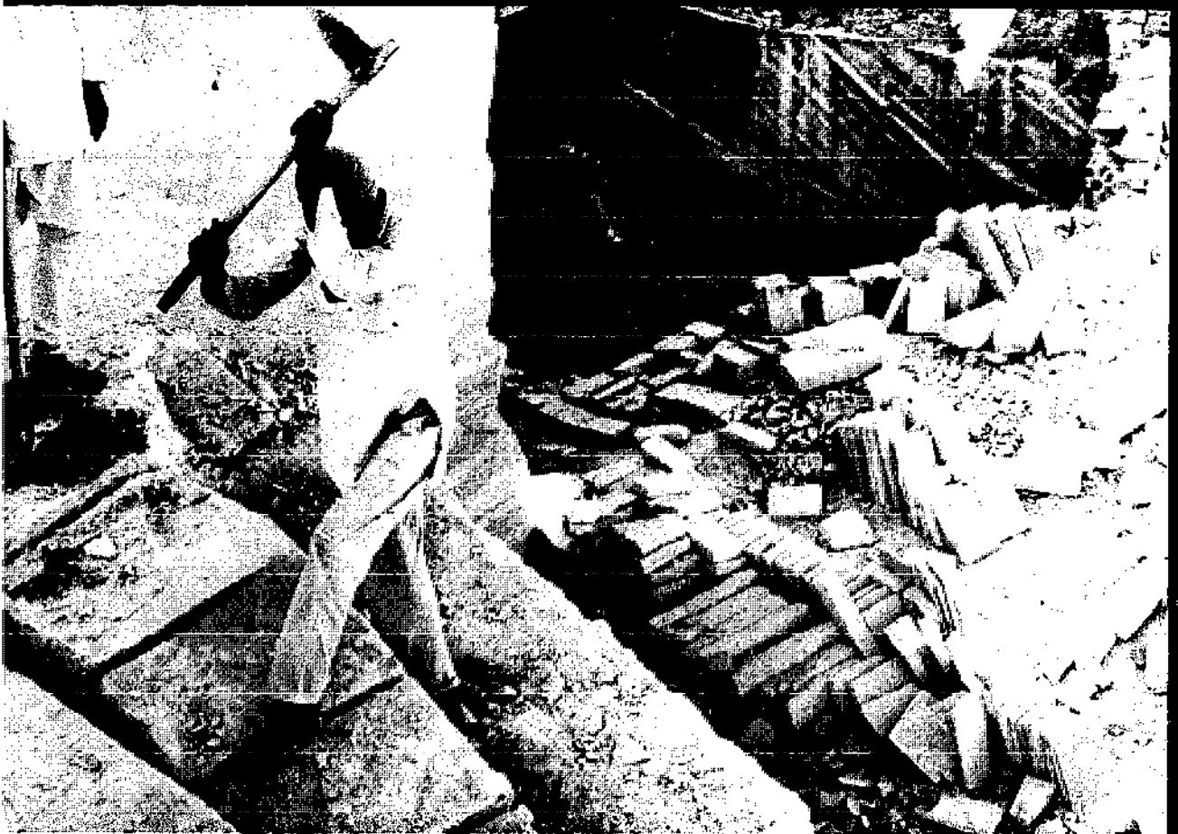
Above: Using a pick axe to split stone in India.
