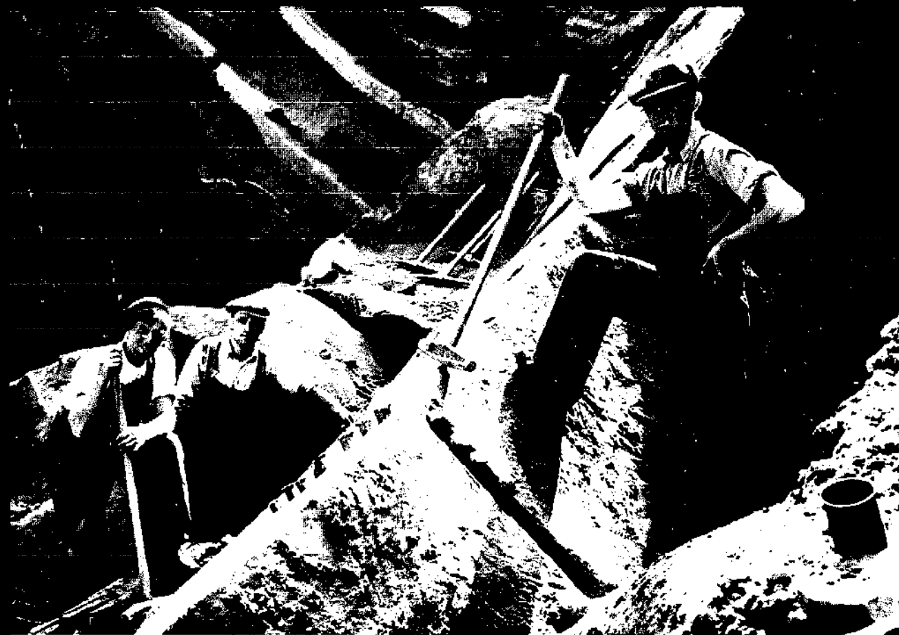
Above: Splitting sandstone by wedge in Scotland
