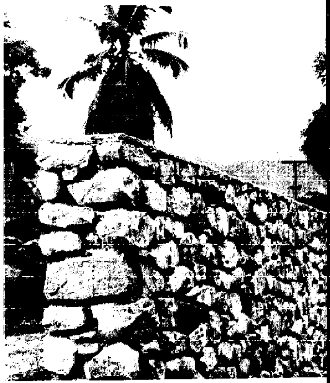
Below (left): Limestone wall of roughly squared field-stones. Below (right): Limestone wall of undressed field-stones held together with mortar.
