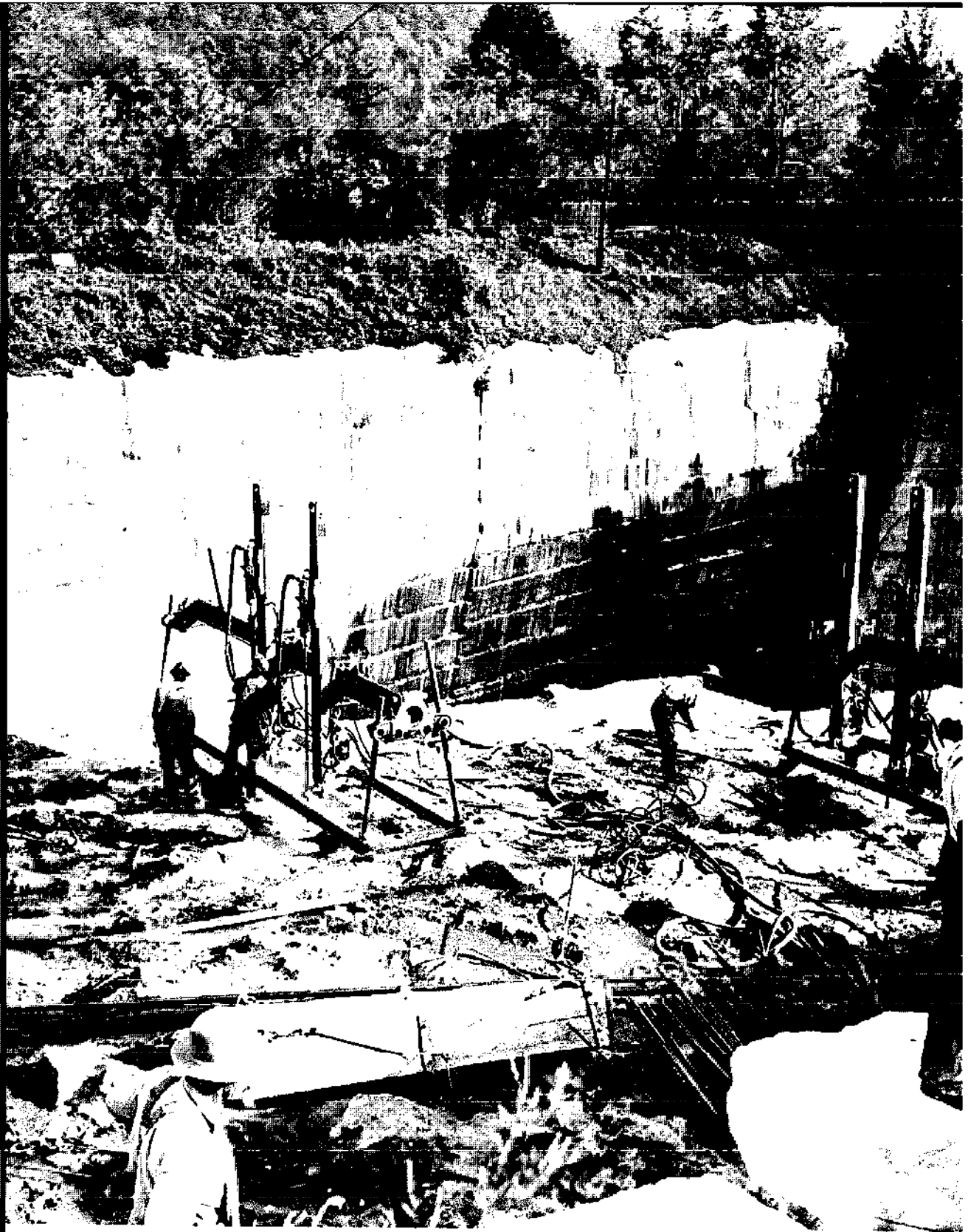
Large wagon drills are mounted on the saddles of quarry bars for accurate drilling at this marble quarry.
