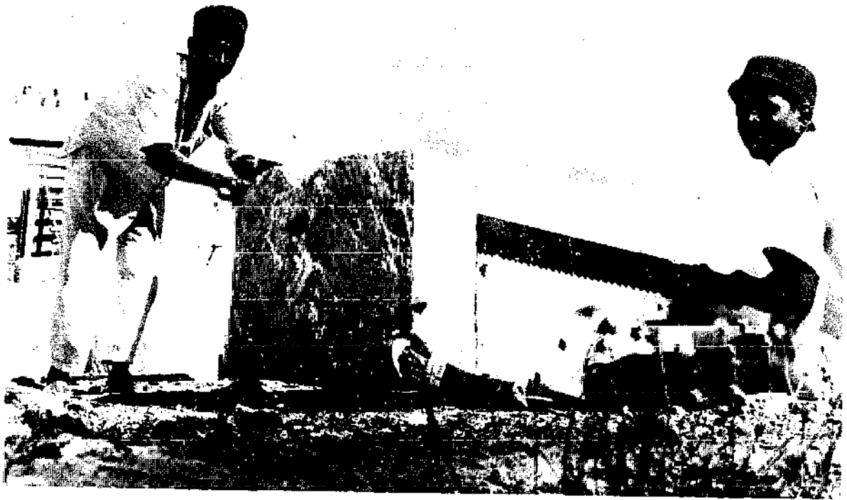
Above: Sawing limestone into building blocks; but industrial blocks have to conform to exact measurements.
