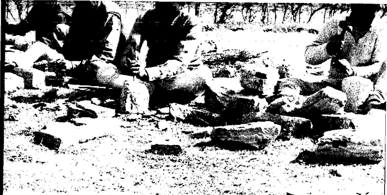
One of the greatest advantages of stone is that it can be shaped using a hammer and chisel (above). Once squared, blocks can be used to build simple buildings, such as this dry-wall dwelling, from Argentina (below).
