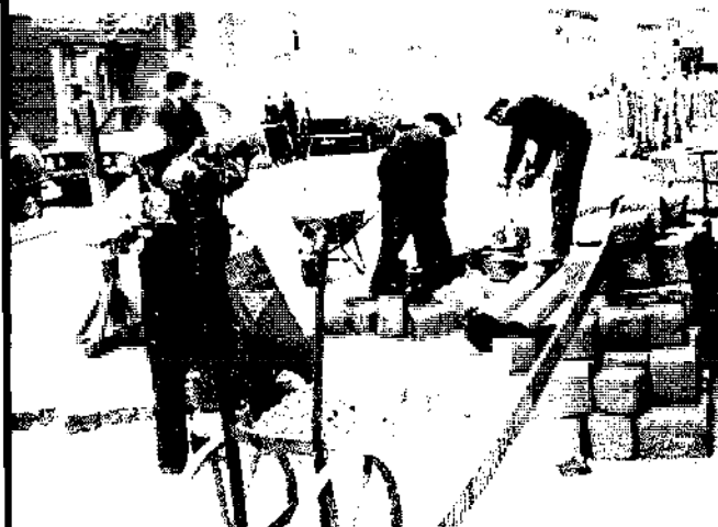
Below: Street pavement under repair using squared granite setts.
