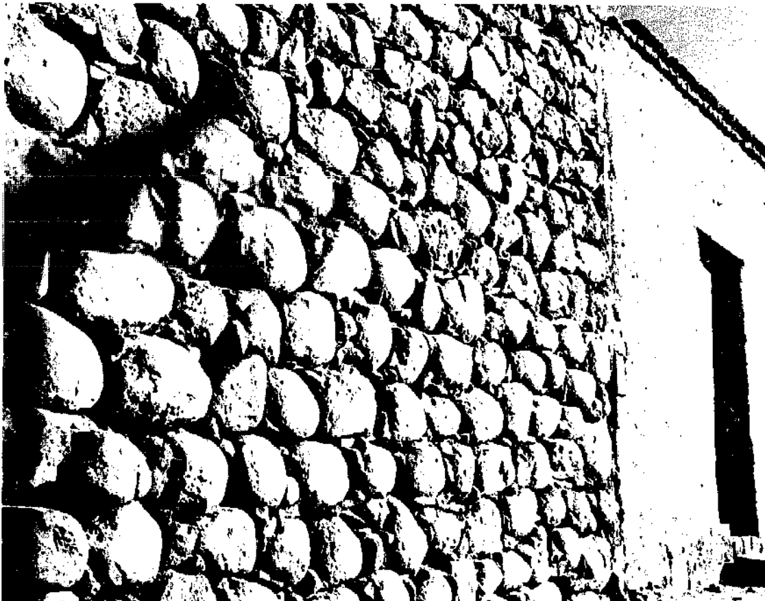
Below: Dry wall made from granite boulders, cobbles, smaller pebbles and stones.
