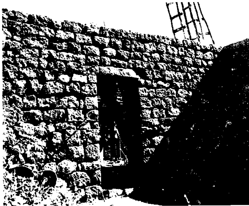
Above: The lintel over this doorway in La Rioja, Argentina, is made from solid granite. Note the stones in the lower courses which are usually larger to increase stability.
