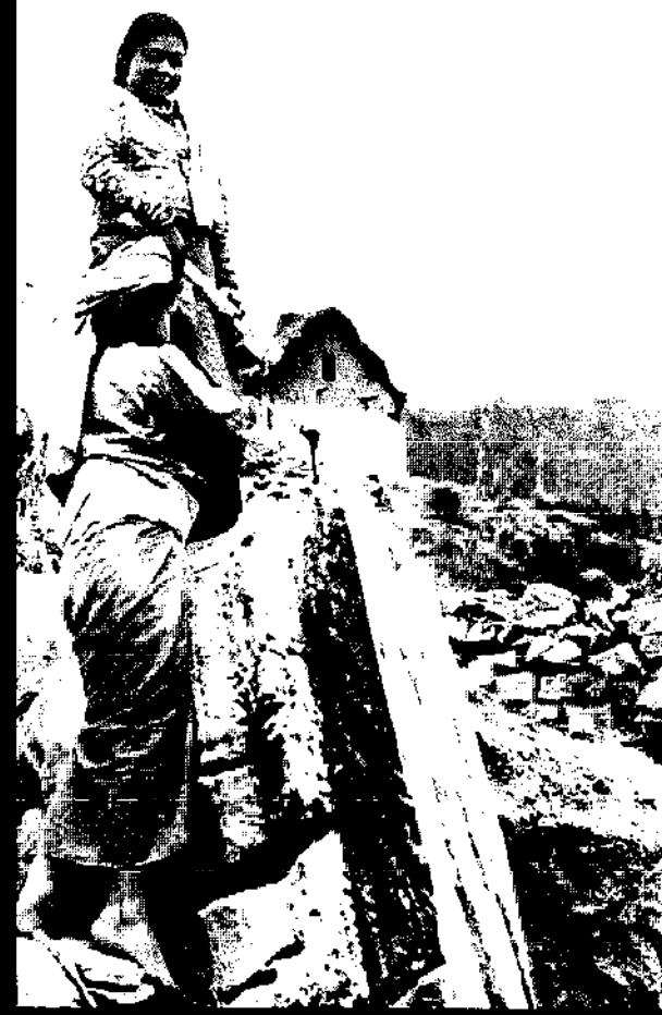
Above: Splitting sandstone by wedge in Scotland
