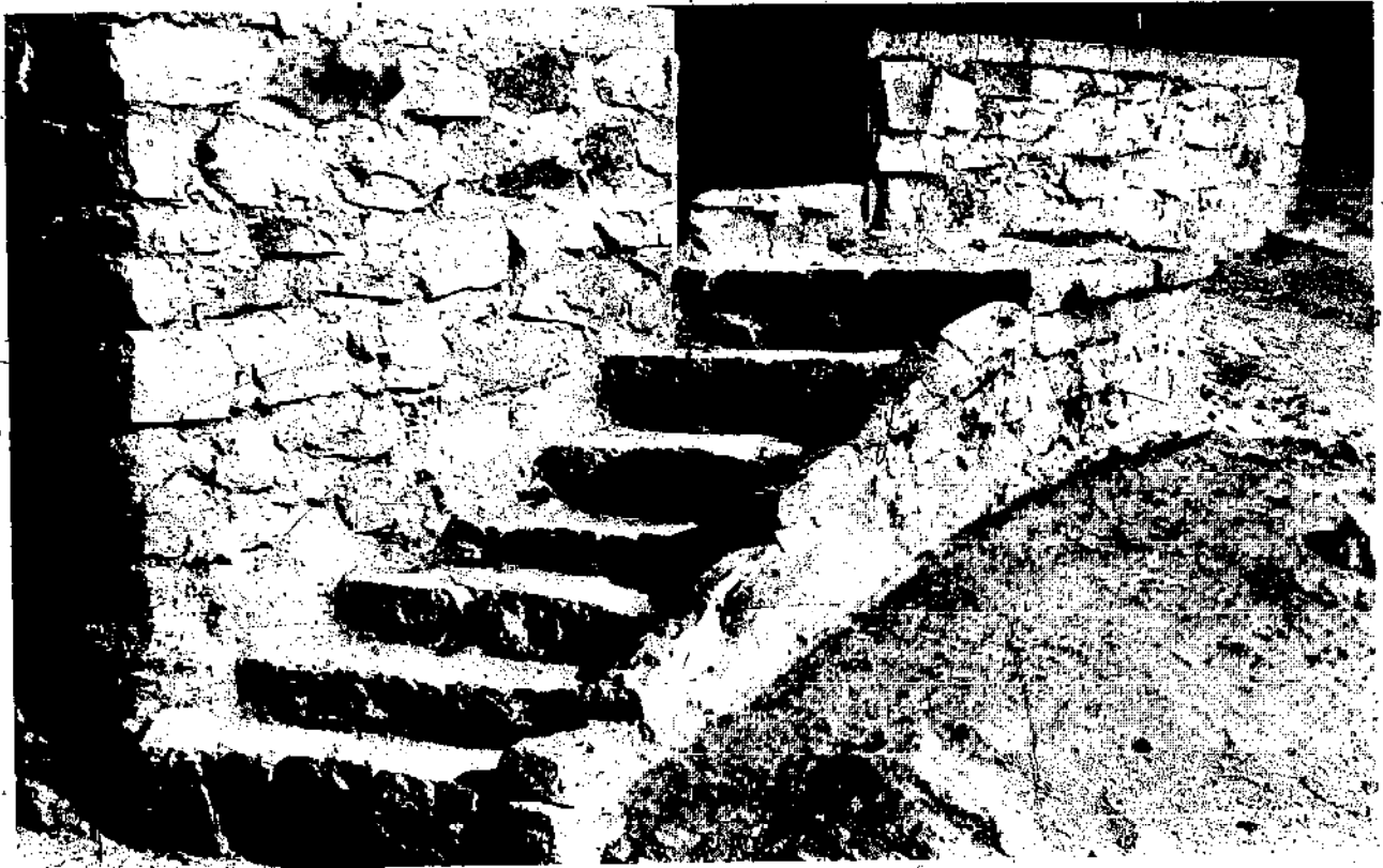
Steps under construction
