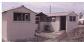
Rebuilding Bam Spring/Summer 2004
