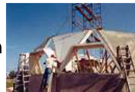
placing a panel into position
