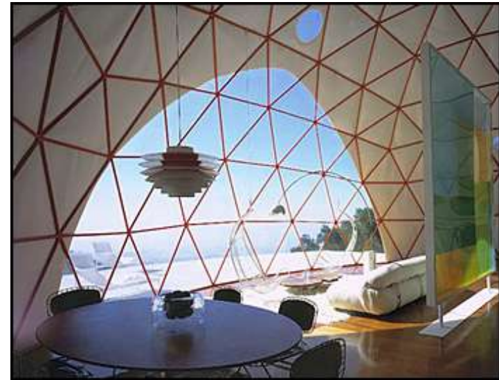
Same dome showing interior. Reflectix allows orange powdercoated frame to show.
