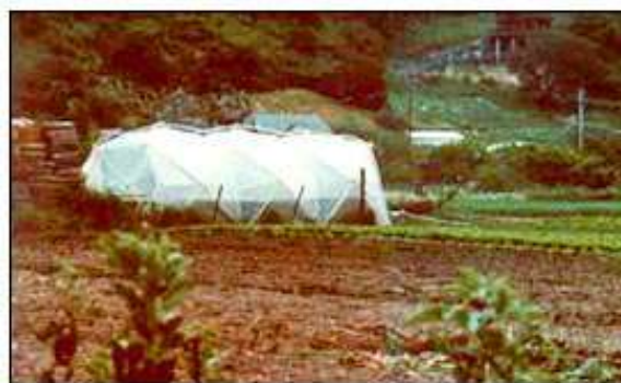
CrystalCave™ 11 made of translucent greenhouse material .
