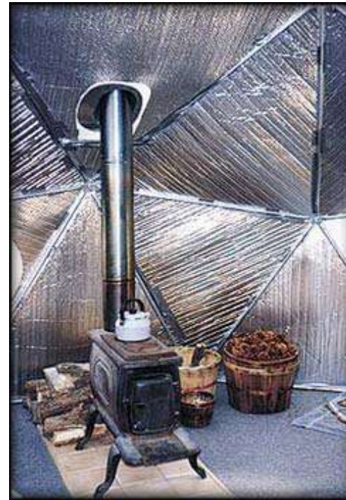
instilation of insulation
