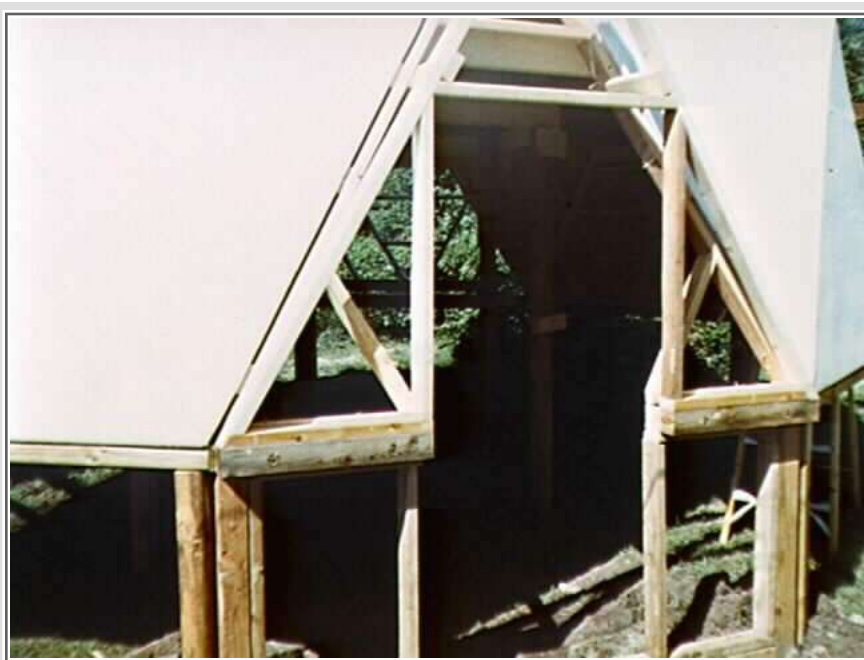
The awning support structure
