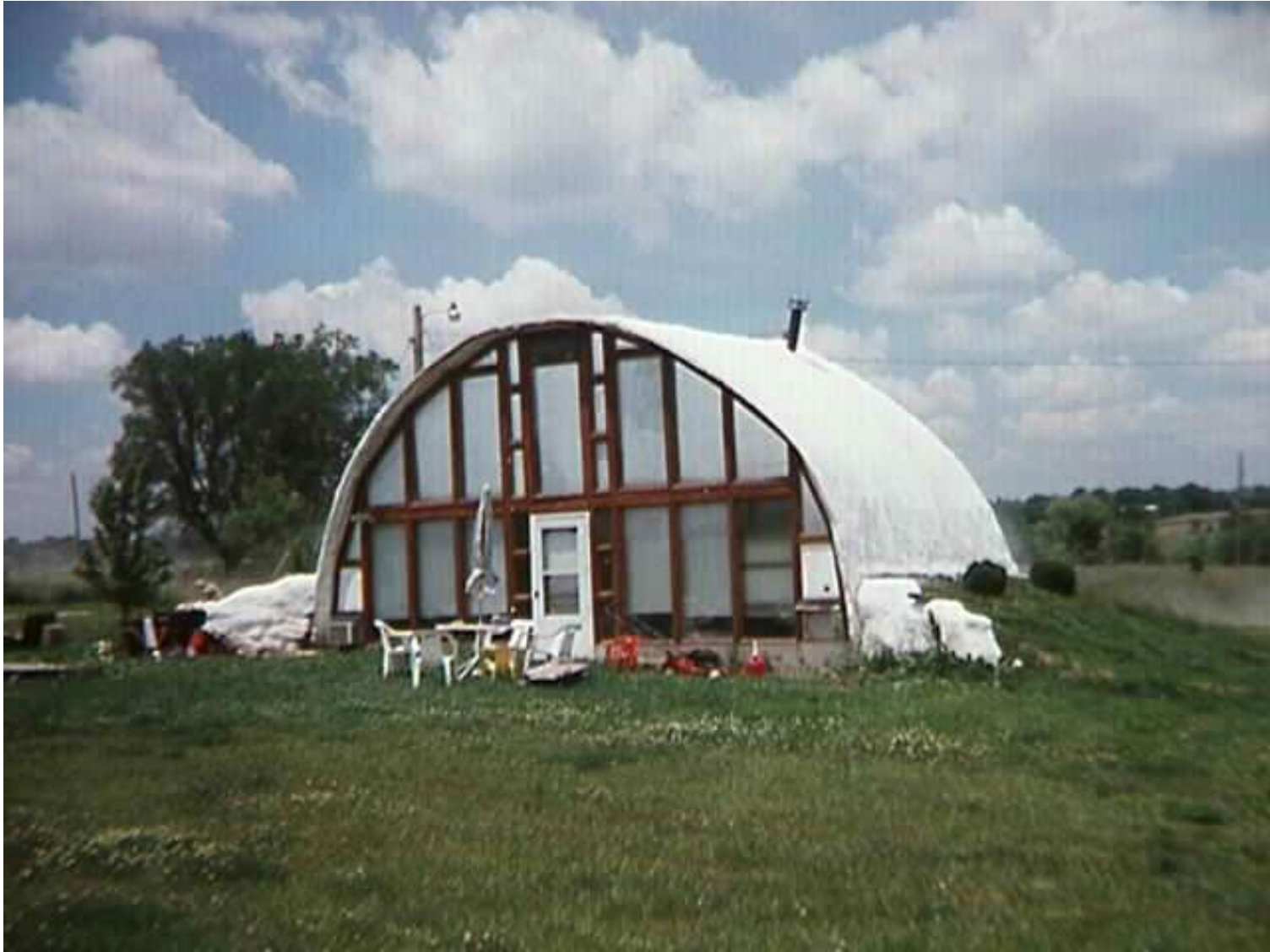
30' Diameter Lightweight Earthcontact Concrete Dome
