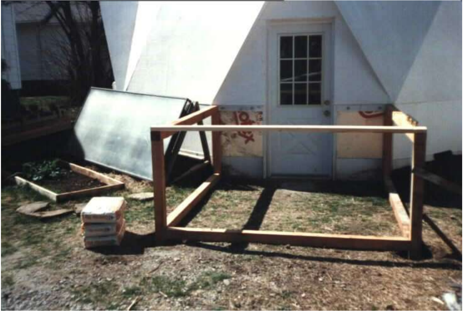
Post & Beam laid being laid out.
