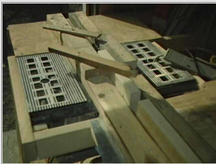
Ripping the predrilled Wedge connector boards
