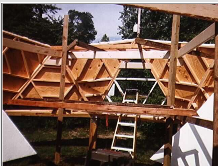
Temporary scaffold used for 2nd level panels
