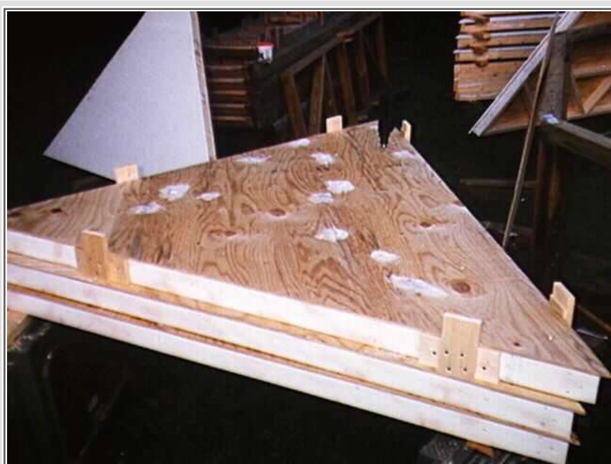
Cleats are used to position sheathing to panels
