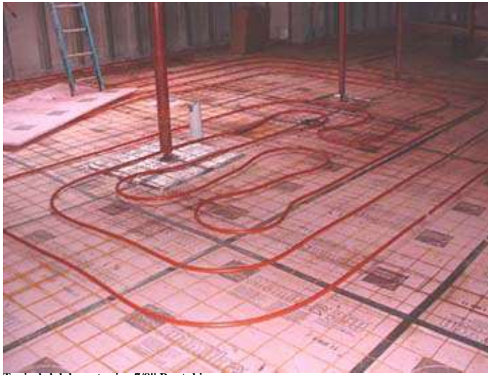
Typical slab layout using 7/8" Pex tubing
