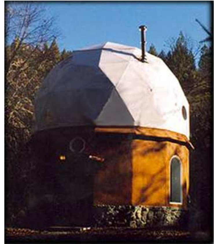
20ft dome as second floor.
