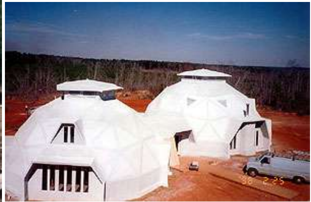
During painting using a latex house paint.
