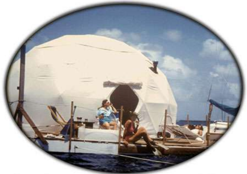
This 20' Dome went through hurricane Andrew in the Florida Keys and was undisturbed by 135 mile an hour winds.
