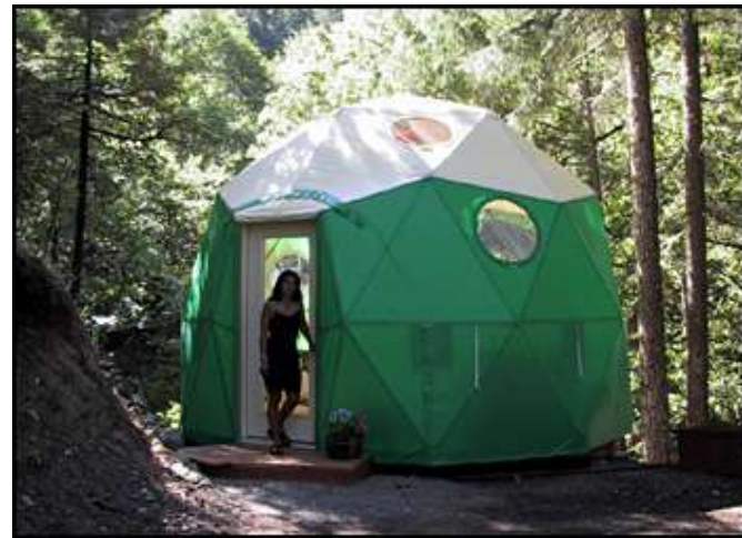
Riser wall allows a pre-hung door option
