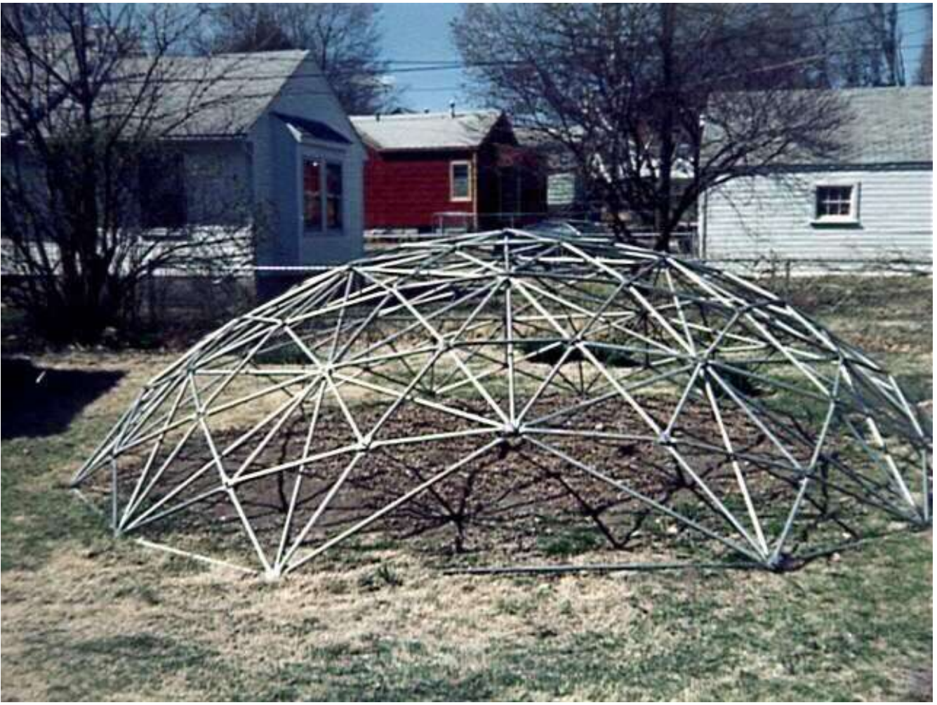
12' Radius-1/5 Compound Geodesic
