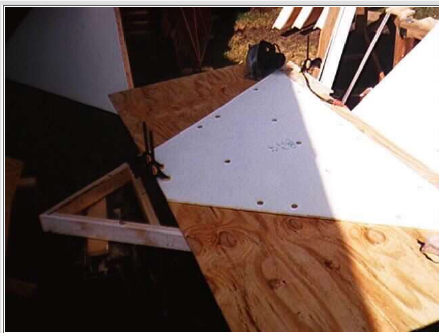
A Pattern is used to cut the plywood sheathing
