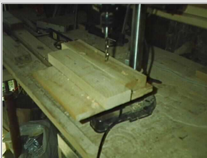
Boards being drilled to make wedge connectors
