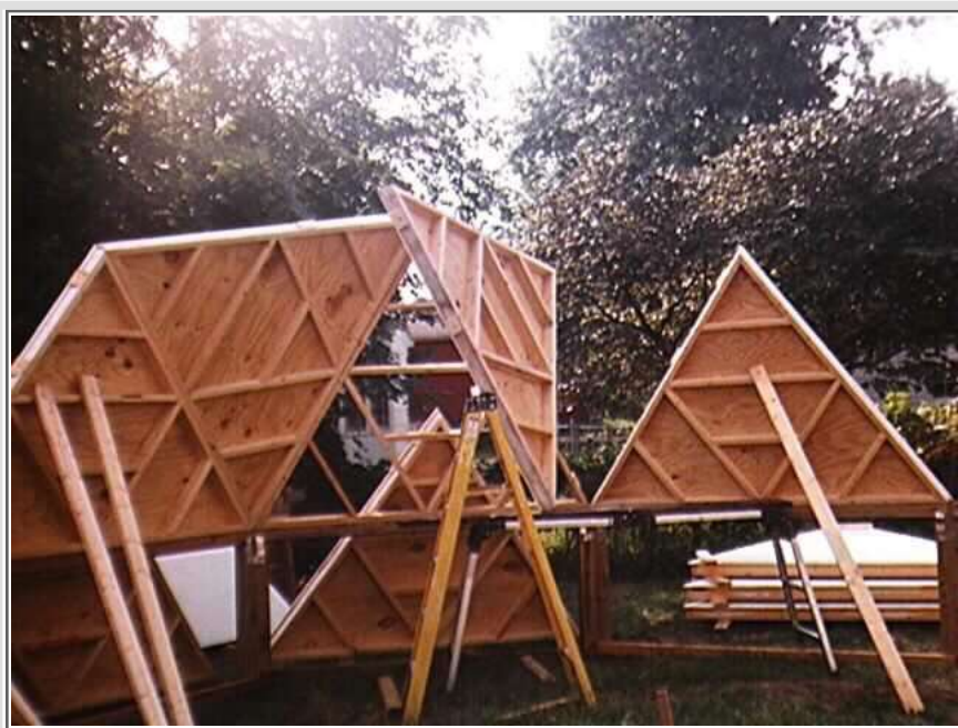
First level panels braced at 10 degree slant
