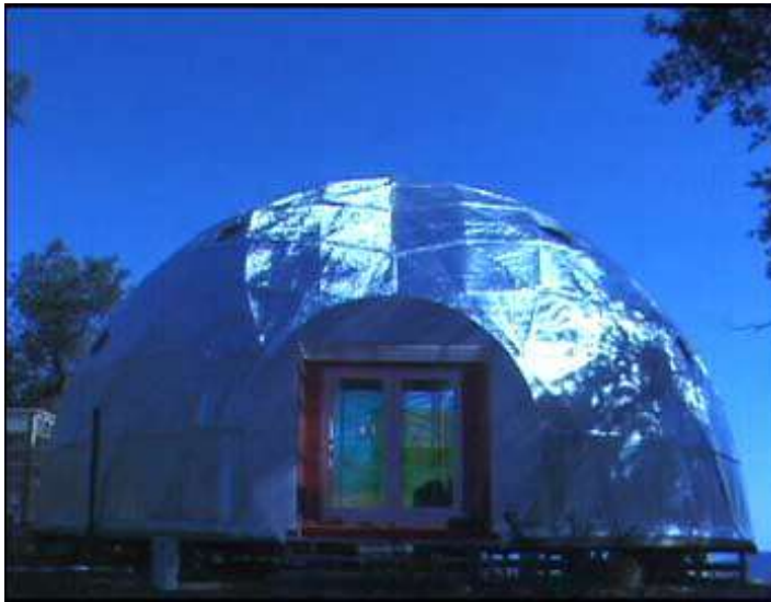
44 ft dome in California with white back Reflectix before canvas was put on.
