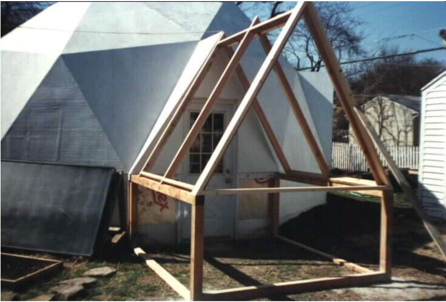
Roof Truss Installed
