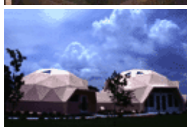
our office complex
