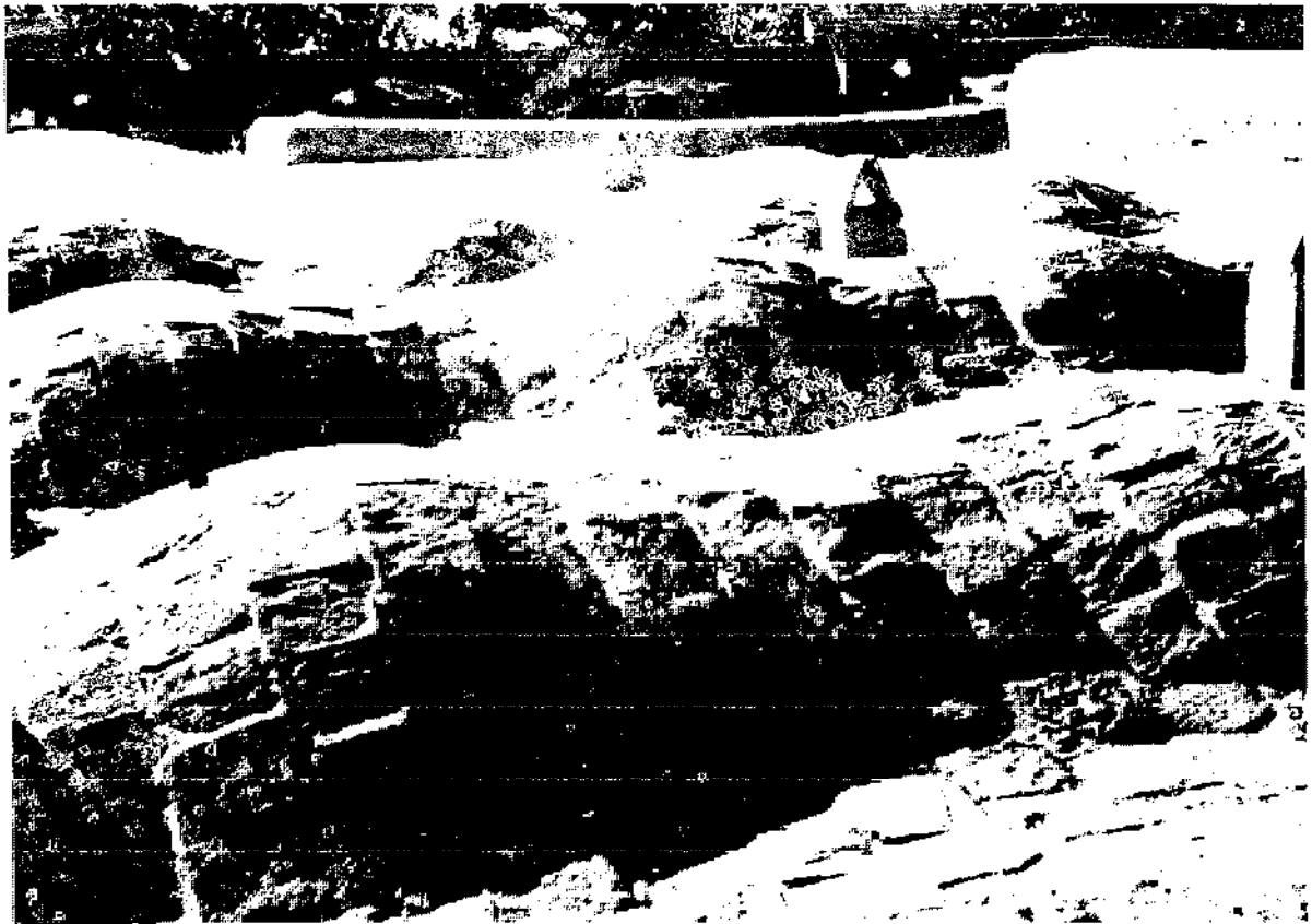
FIG. 5.25. Doubly curved mud-vault roof, Iran.
