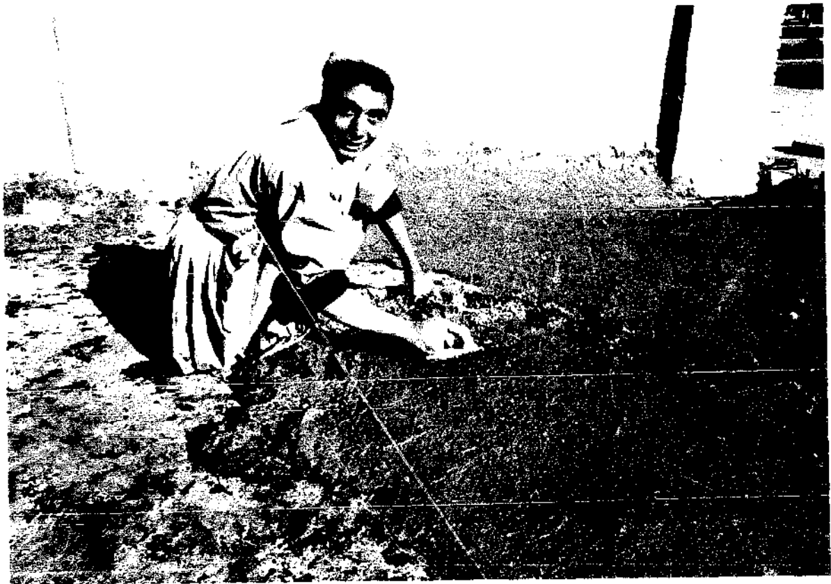
In Herat, Afghanistan, a mud-straw mixture is mixed on the ground and then carried up to resurface the roof of a house. Photos: Sean Sprague
