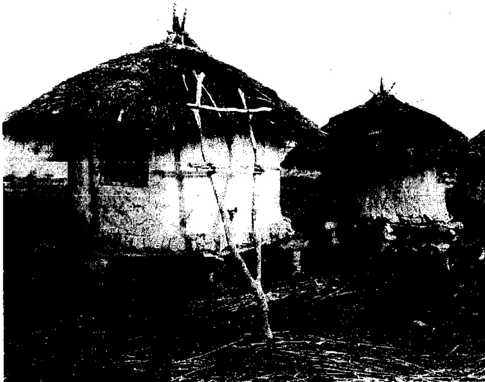
Mali mud granaries are protected from rain by an overhanging grass roof, and stand off the ground to avoid floods and rising damp. (Note the simple ladder for repairing the roof.)
