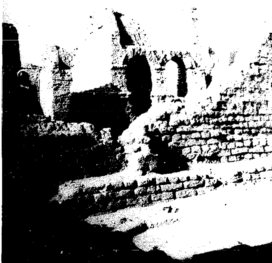
10th century Coptic church in Aswan, Egypt. Modern architect Hasan Fathy uses the ancient technique of mud vaults to help solve the housing needs of today.
