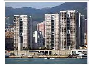
Clague Garden Estate, a public housing estate in Tsuen Wan
