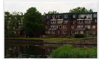
1970s council housing in Haringey, North London.
