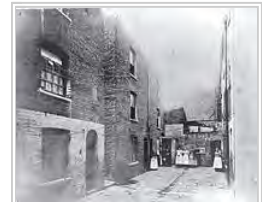
Boundary Street 1890, three years later, the London County Council began slum clearance
