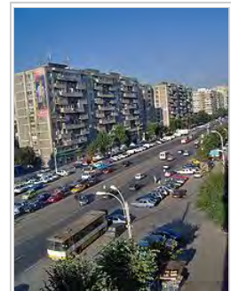
Government built housing in Bucharest, Romania
