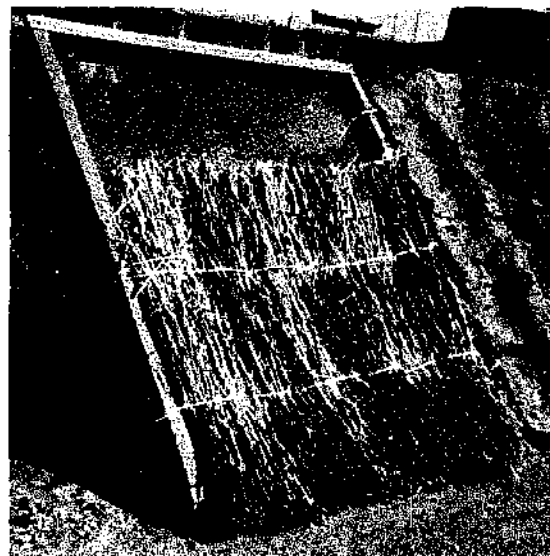
Fig. 6.10 On chicken-wire substructure, first layer of pajón bundles, each layer receiving a coat of bitumen emulsion waterproofing before attachment of next layer.
