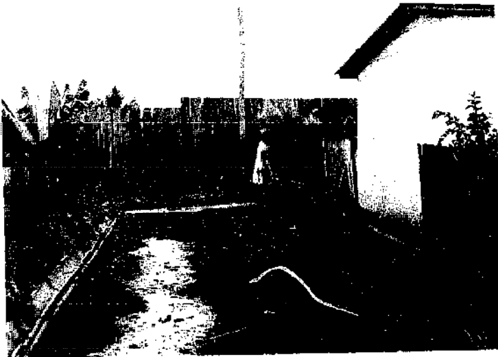
Ponds are formed by liquids leaking from the sewerage system
