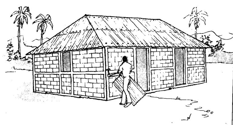
Fasten each galvanized sheet securely to the roof. Use a minimum of 12 nails for each sheet.
