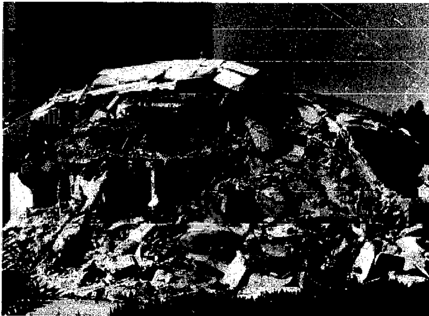
In both the southern Italian and Algerian (El Asnam), earthquakes of 1980 there was widespread damage to recently built, reinforced concrete buildings, despite the existence of seismic building codes. This highlights the need for improved training of builders and the need for effective enforcement of building codes.
