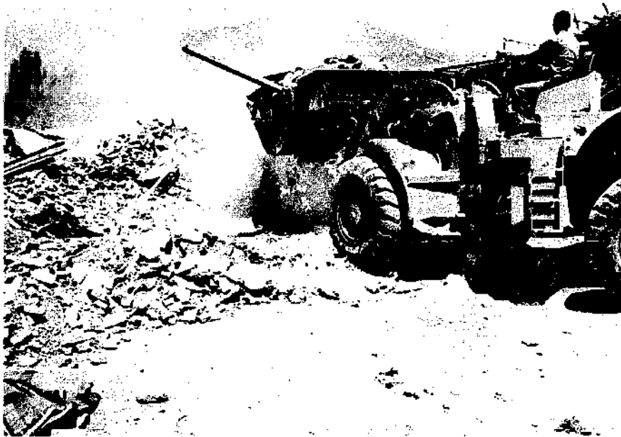
The mechanized clearance of rubble (seen here after the Guatemalan earthquake of 1976) can remove vital building materials which are capable of being recycled for new construction, such as the beam projecting from the front of the bulldozer.
