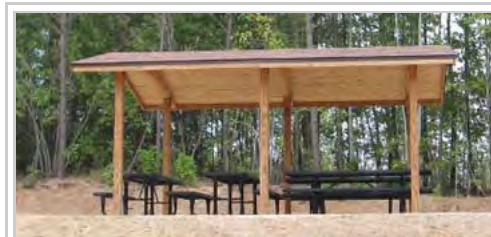
Northeast Park Picnic shelter
