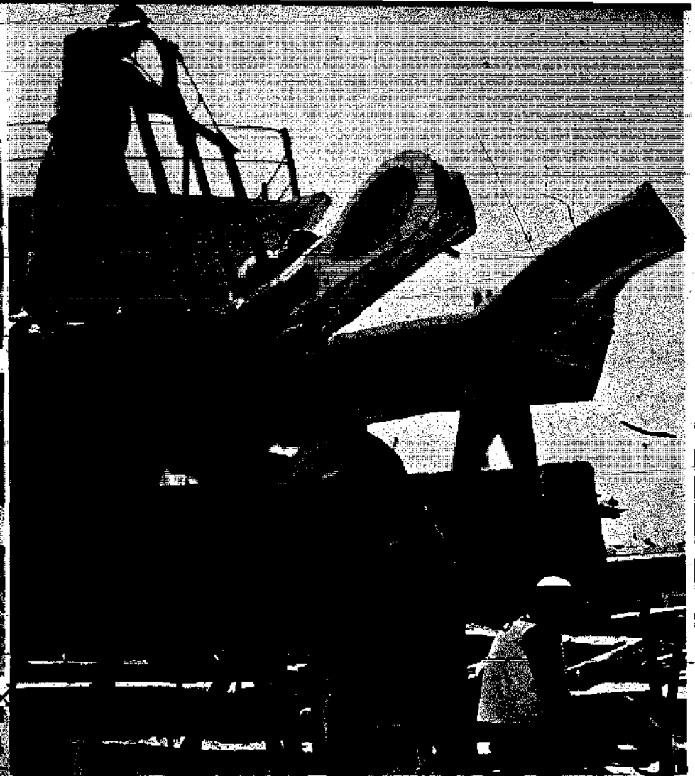
Egyptian boat builders use natural bend of trees to cut boat beams, using log's grain for maximum strength.
