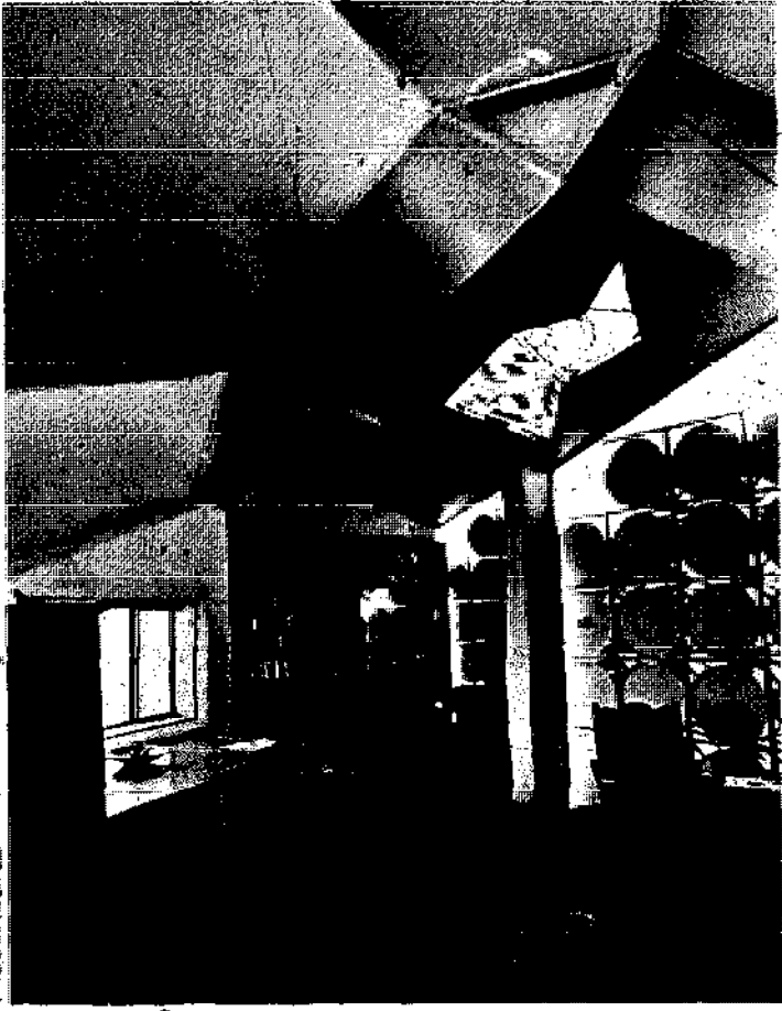
The house consists of 10 exploded rhombic dodecahedra stretched and fused to form the different sized rooms...is heated by the four drum walls, four skylights and two small wood stoves.
