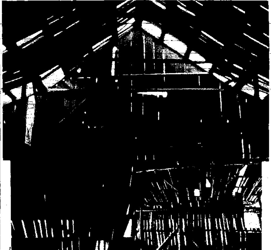
100 year old Barn near Santa Rosa, Calif. Redwood saplings were nailed together. Nails were added off on top and bottom, but posts and braces were left tight.
