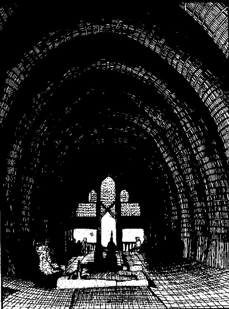
The building above is of a mudbi built by the Ma'dan or Marshmen of Southern Iraq. It is a 6,000 year old building technique, involving use of the giant reed ( Jragmites communis ) that grows to a height of 20' along the lower Tigris and Euphrates. It is bound into bundles, which are then stuck into the ground opposite each other in two rows. A man then climbs onto a reed tripod, and as others pull the tops down, binds them together. When the arches are in place, horizontal ribbing is fastened, then mats tied in place. This structure is a restaurant outside Baghdad, Iraq.
