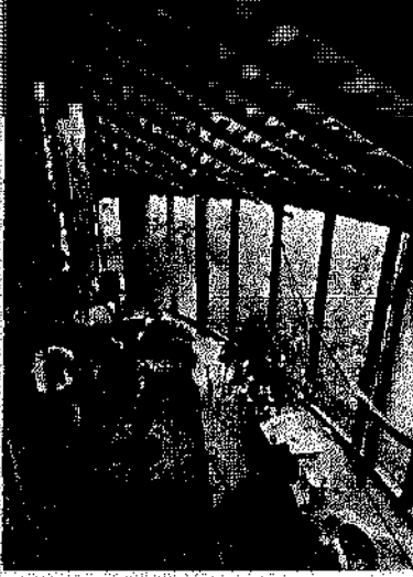
Val's own house. The roof is framed with 2x4 rafters on 1200 Joist centers, with 1x4 stripping spaced 4" apart over the rafters. The underside of the shingle roof is exposed between the stripping. The earring ridge and plate beams are
