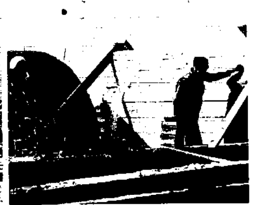
Chorfa, vaulted structures in Tunisia. Originally as grain storage by keys for nomad tribes, now being used for living. Making walls
