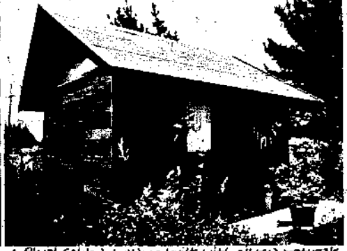
A 8'x15' Gabled building built with all used materials
