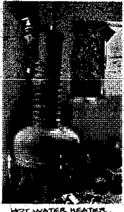
HOT WATER HEATER.
