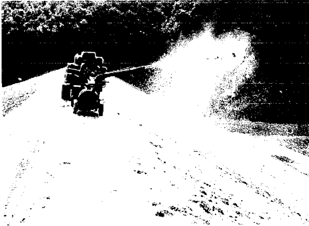
Fig. 13-12. Mulching machine operating on new fill.
