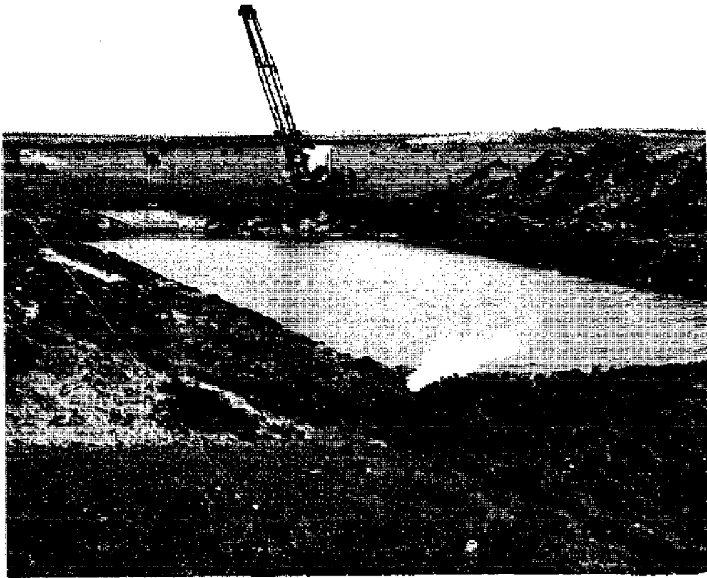
Fig. 11-17. Excavating a pond with a dragline.
