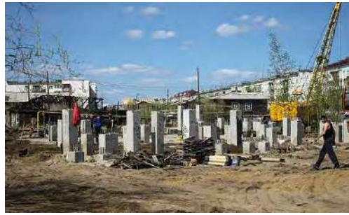
Pile foundations in Yakutsk, a city underlain with continuous permafrost.
