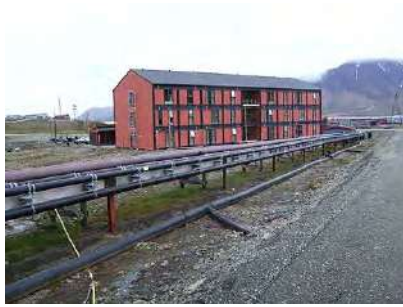
Above-ground utility lines in a permafrost zone avoid thawing of ground.
