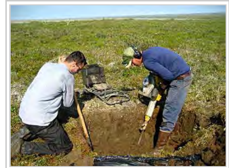
Excavating ice-rich permafrost with a jackhammer in Alaska.
