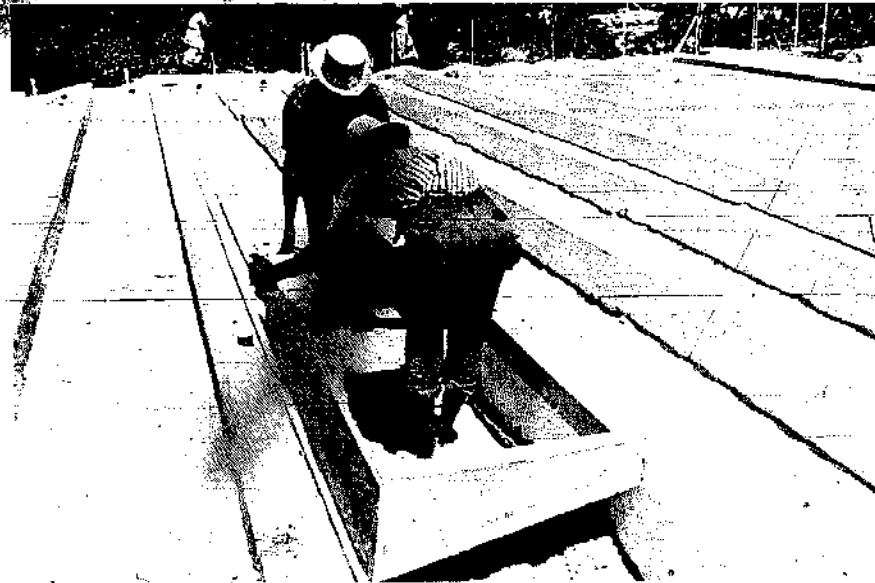
Fig 6: Finished curb and end walls with basin fill. The wooden frame is the guide used in levelling the basin fill in each of the twelve 6 foot long ponds that form one bay
