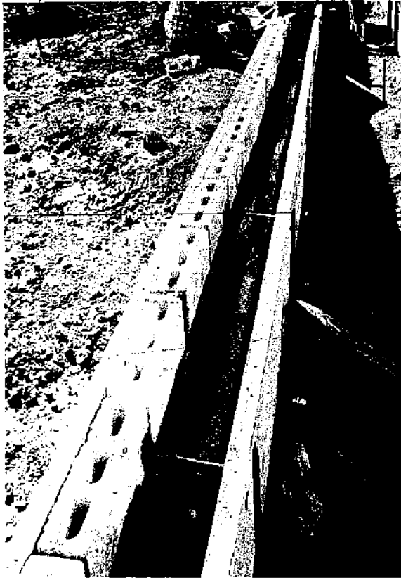
Fig 3: General view of partially completed curb wall, illustrating wood form work, rough gutters and concrete blocks. Note that at each tie wire, a bottom portion of the concrete block had to be chipped away. As noted in text, subsequent courses of concrete blocks were placed after tie wires had been removed
