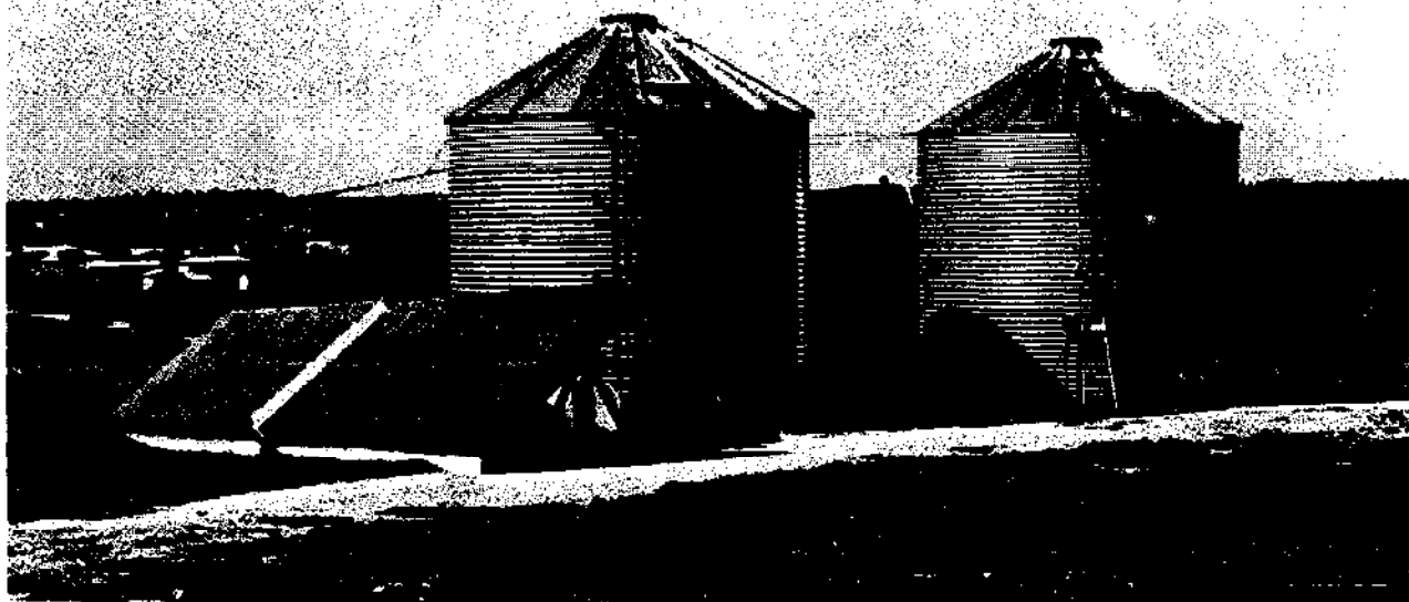
Figure 3 Portable Flat-Plate Solar System used in corn drying experiment, located at U.S. Grain Marketing Research Center, Manhattan, Kansas
