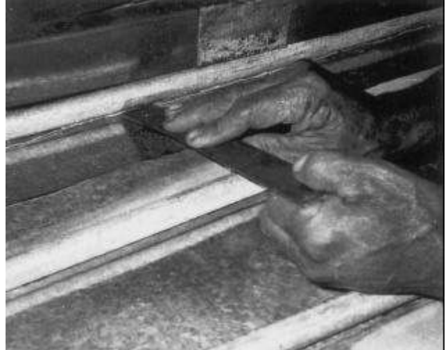
2: Press the strips firmly under the pipe.
