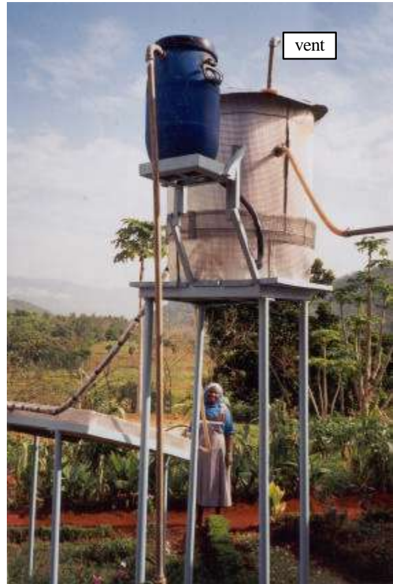
The vent on top of the storage tank should not choke.
