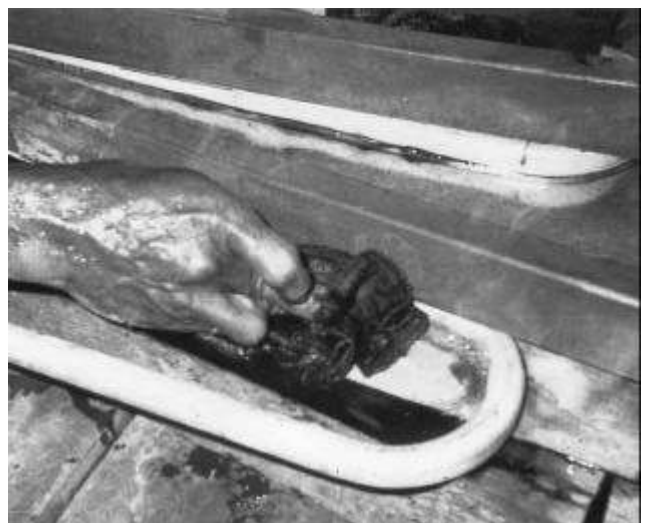
5: Then cool down the solder joint of pipe and sheet with damp cloths and next to remove the superfluous soldering flux.
