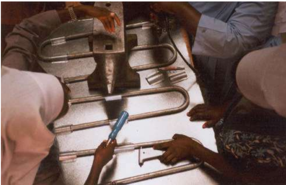
Drilling holes through the metal saddles and metal sheet.
