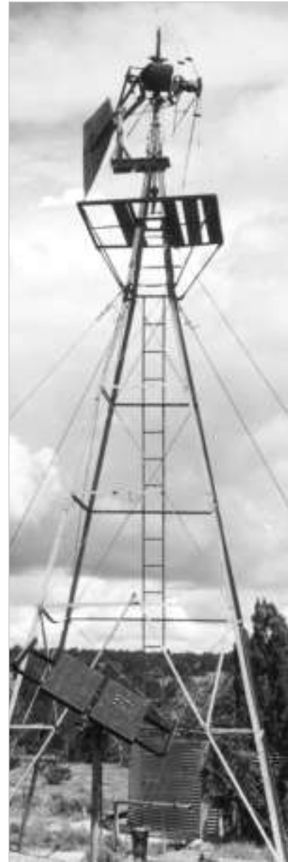
The well under this dead windmill has been brought back to life by a solar submersible pump powered by a 120-watt array.
