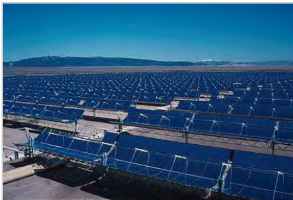
Part of the 354 MW Solar Energy Generating Systems (SEGS) parabolic trough solar complex in northern San Bernardino County, California
