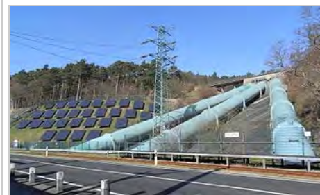
Pumped-storage hydroelectricity (PSH). This facility in Geesthacht, Germany, also includes a solar array.
