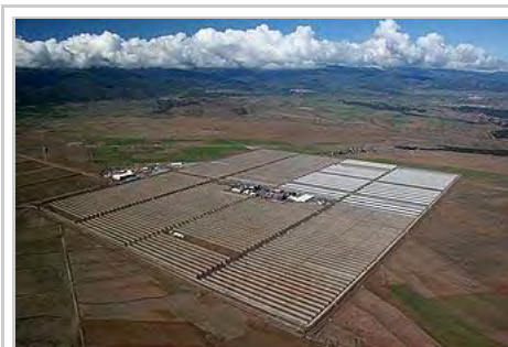
Thermal energy storage. The Andasol CSP plant uses tanks of molten salt to store solar energy.
