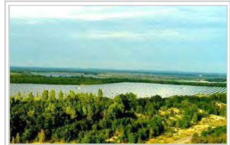
Part of the Senftenberg Solarpark, a solar photovoltaic power plant located on former open-pit mining areas close to the city of Senftenberg, in Eastern Germany. The 78 MW Phase 1 of the plant was completed within three months.
