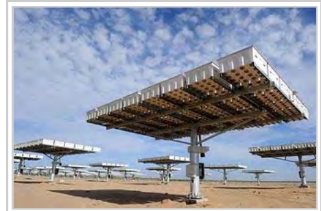
CPV modules on dual axis solar trackers in Golmud, China
