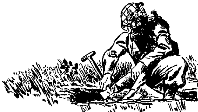
SPOIL BEING REMOVED CORRECTLY
