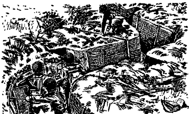
Figure 12. Installing burlap and chicken-wire revetment.
