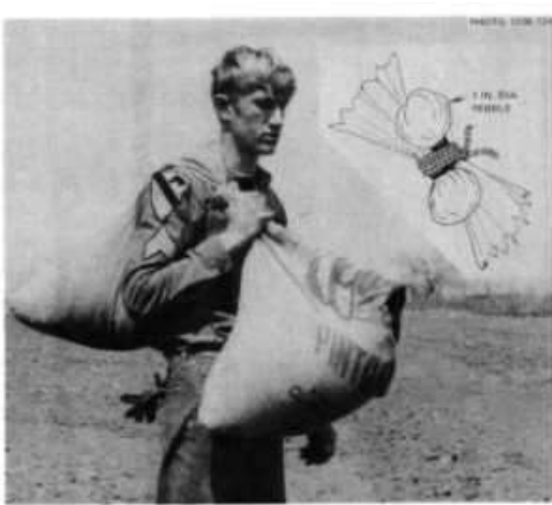
Fig. 8.1. Carrying 80 pounds of water in two burlap bags, each lined with two larger plastic trash bags, one inside the other. (Photograph)
