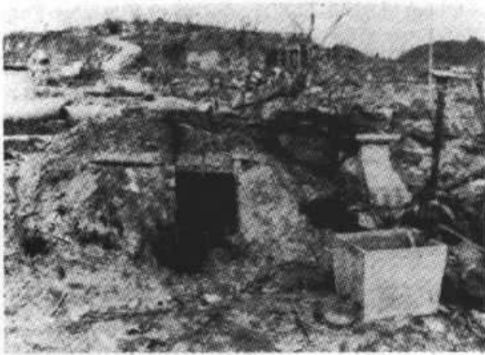
Fig. 1.5. Undamaged earth-covered family shelter in Nagasaki.
