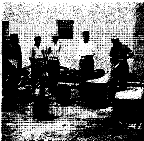
FIGURE 20. - Slaked lime can be made correctly in iron drums.
