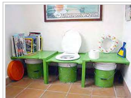
Bucket toilet with spare buckets stored on either side.
