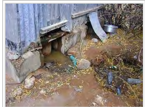
Access point for buckets of a bucket toilet in North Eastern Province, Kenya (near Wajir)
