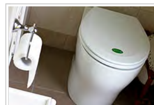
This is the pedestal for a split-system composting toilet where collection/treatment chambers are located below the bathroom floor.
