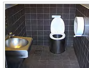
Public composting toilet at a highway rest facility in Sweden
