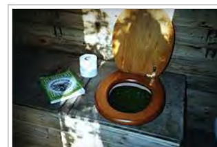
Inexpensive do-it-yourself compost toilet at Dial House, Essex, England, utilizing an old desk as the toilet unit.
