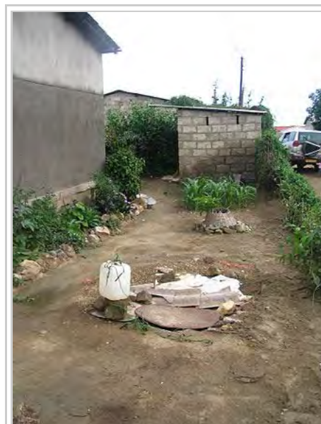
Common problem: groundwater well (forefront) is in close proximity to the pit latrine (brick building at the back) in Lusaka, Zambia
