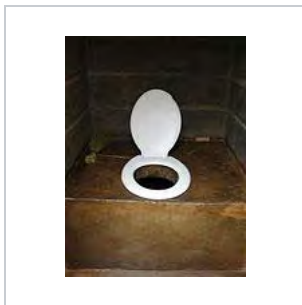
Pit latrine from the inside at a household near Maseru, Lesotho (same toilet as shown left from the outside).
