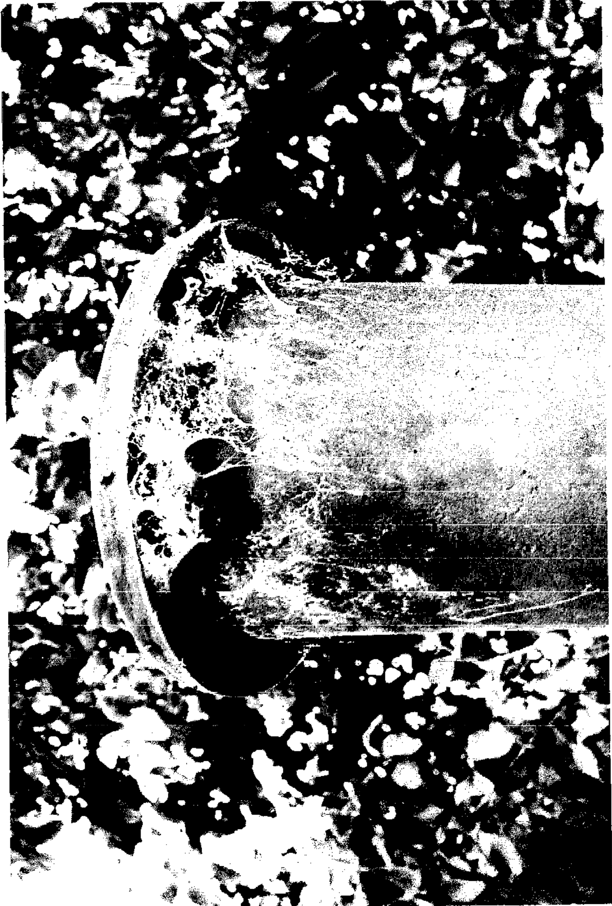
Figure 6: Cobwebs at the top of a vent pipe.
