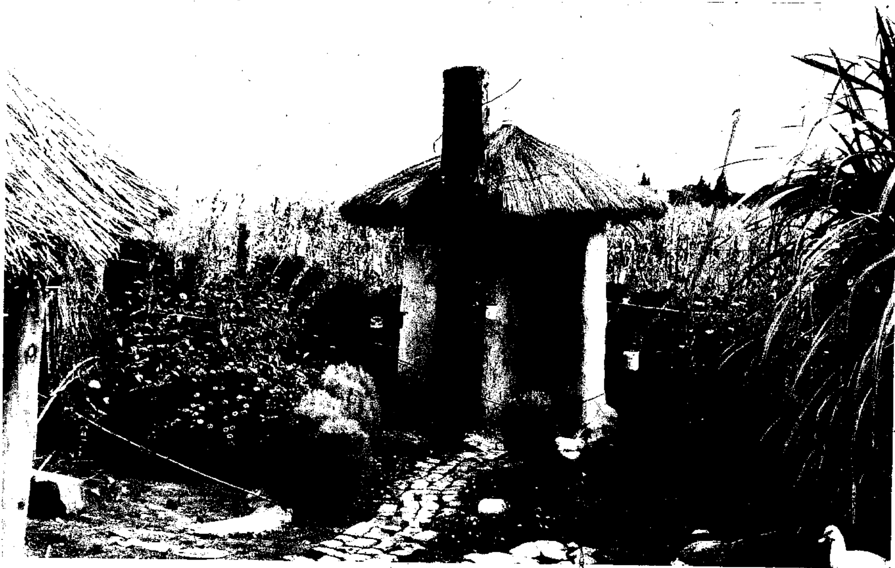
Figure 10: Mud and wattle spiral VIP latrine.
