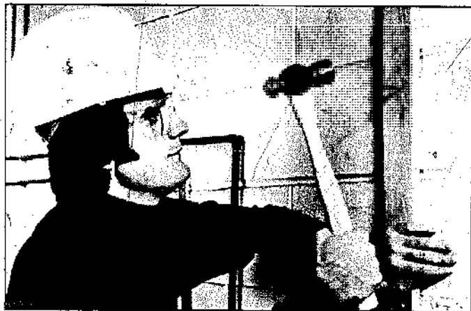
Use a heavy ball-peen hammer for driving special hardened nails into masonry. Note the hard hat and the safety goggles. Hand Tools Institute Photo.
