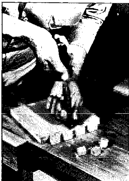
Outline intricate cuts with a knife or coping saw and clean with a chisel. Take slight cuts and be sure the chisel is SHARP.
