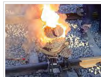
A thermite weld in progress.
