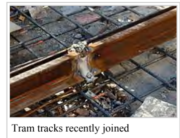
Tram tracks being joined
